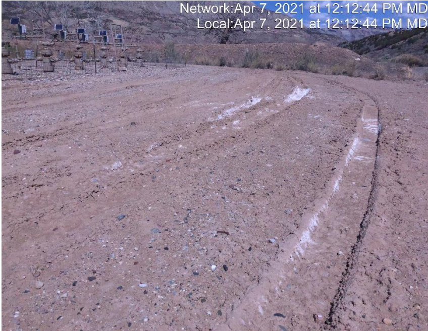
Photo #3394 Location lacks stabilization.
