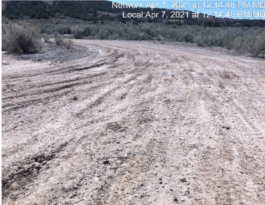
Photo #3396 No form of tracking control at entrance to location.
