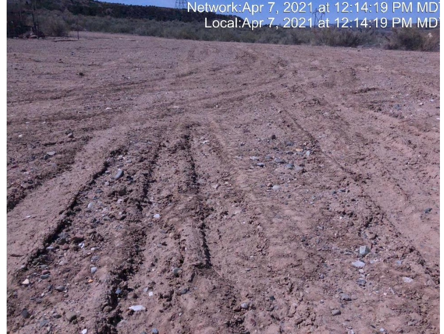
Photo #3395 Location lacks stabilization.
