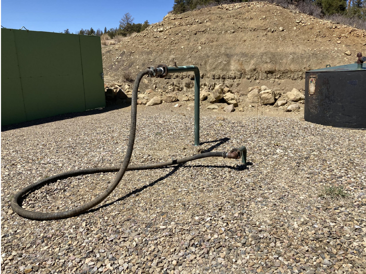
PHOTO 6: THE RISER'S ARE ACTUALLY A LOW PRESURE BY-PASS THAT ARE IN USE. EACH RISER WAS LABELED AS TO IT'S FUNCTION.
