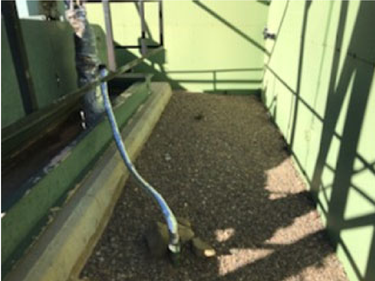
PHOTO 4: THE IMPACTED SOIL NEAR THE PUMPING UNIT WAS REMOVED AND PROPERLY DISPOSED IN ACCORDANCE WITH THE OGRIS OPERATING WASTE MANAGEMENT PLAN.
