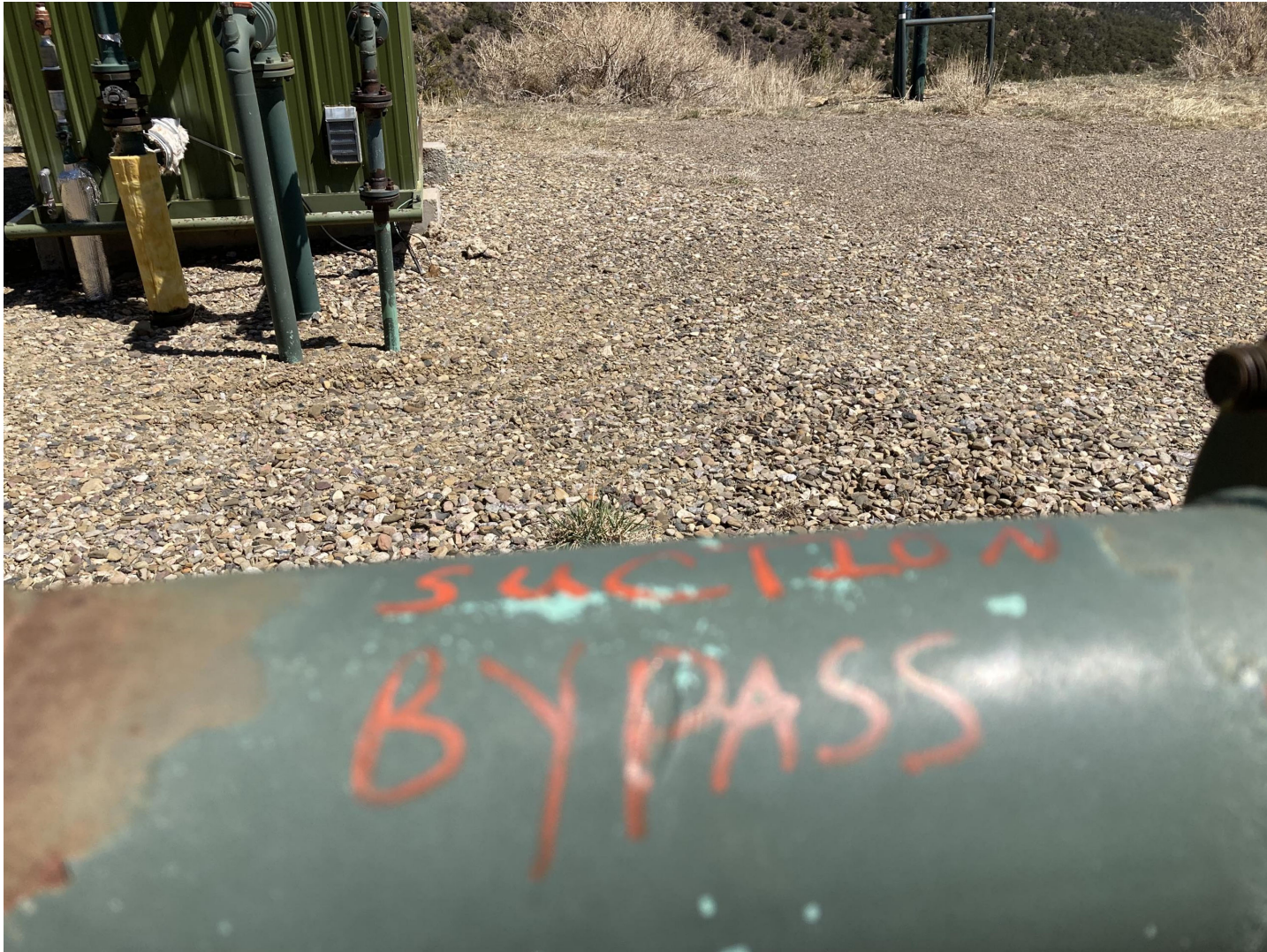
PHOTO 8: THE RISER'S ARE ACTUALLY A LOW PRESURE BY-PASS THAT ARE IN USE. EACH RISER WAS LABELED AS TO IT'S FUNCTION.
