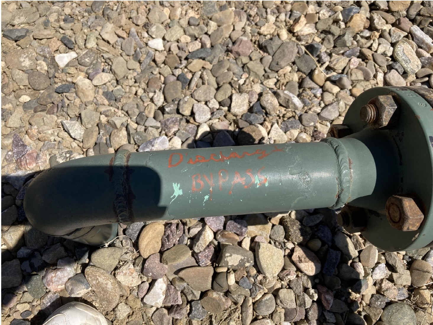
PHOTO 7: THE RISER'S ARE ACTUALLY A LOW PRESURE BY-PASS THAT ARE IN USE. EACH RISER WAS LABELED AS TO IT'S FUNCTION.
