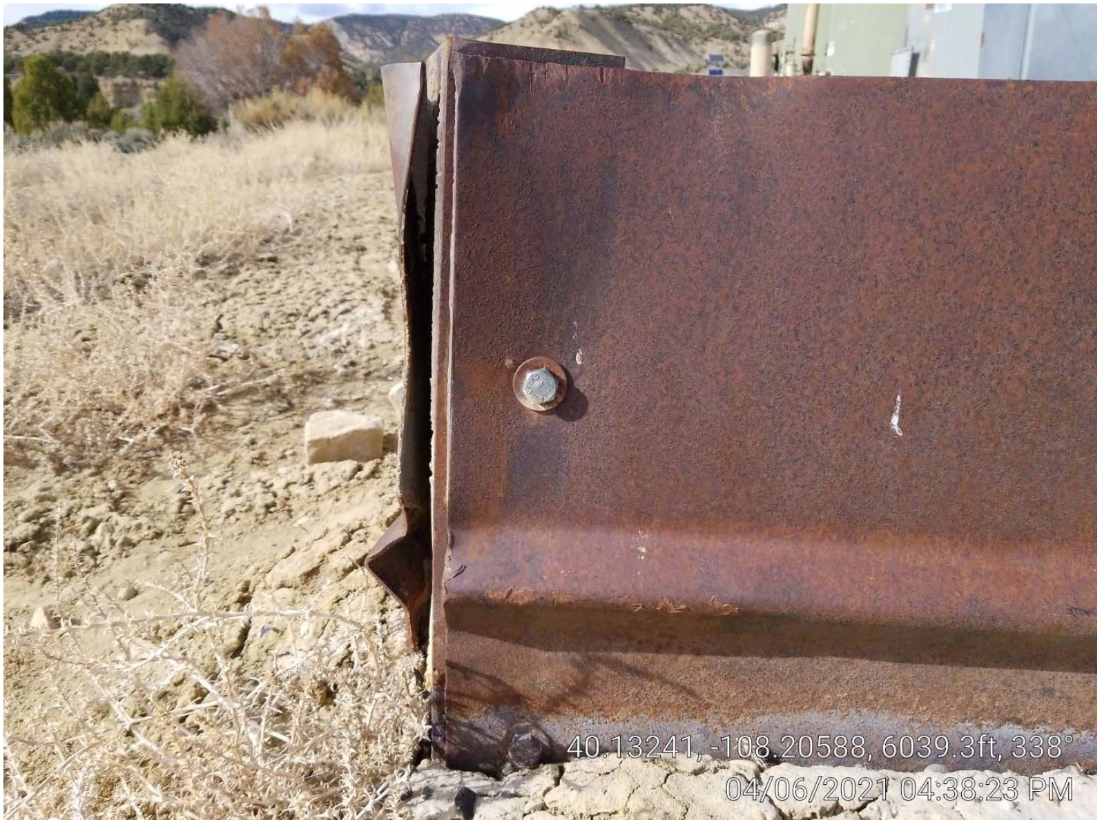
Photo 7. Gap in tank secondary containment.
