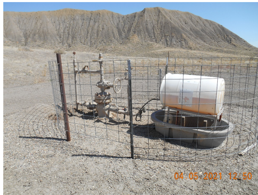
Wellhead with fence. Secondary containment of chemicals.
