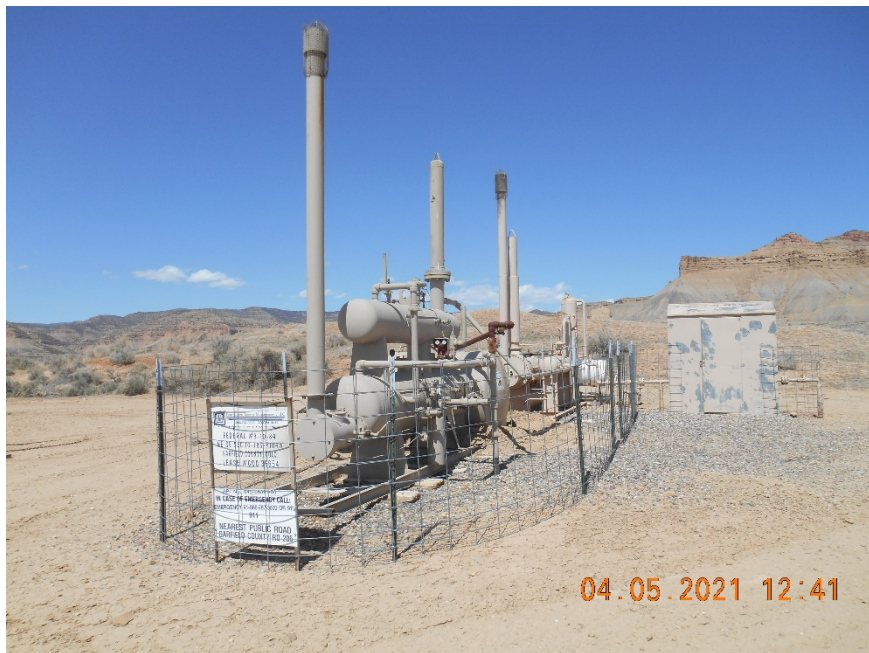
Separators with blowdown tank, Meter housing and sign.
