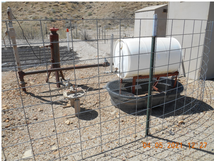
Secondary containment of chemicals. Contents and NFPA labels faded/unreadable.
