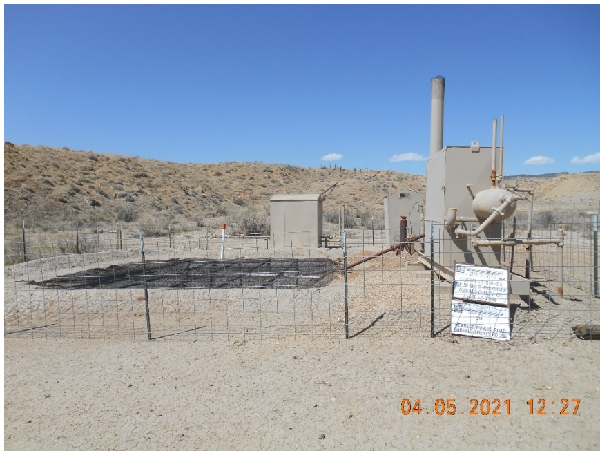
Separator and Meter housings with blowdown pit. Location sign.
