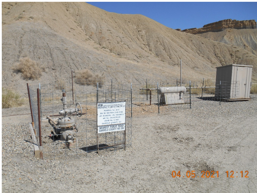
Wellhead with fence & sign. Separator and Meter housing.
