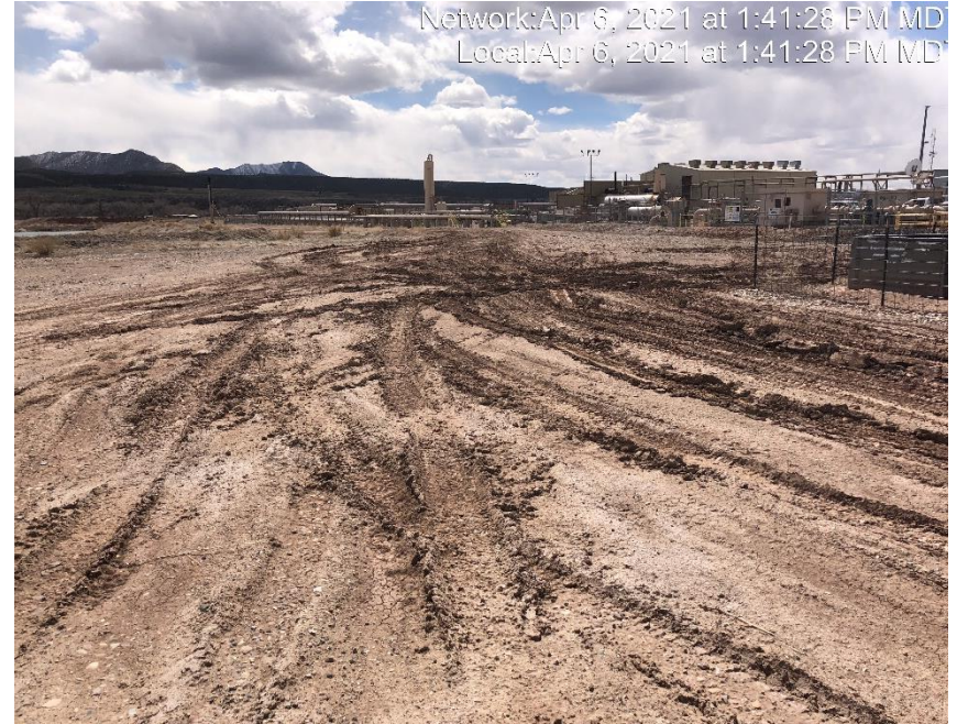
Photo #3388 No form of tracking control at entrance to location.
