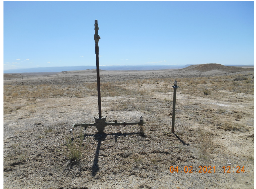
Wellhead Temporarily Abandoned.
