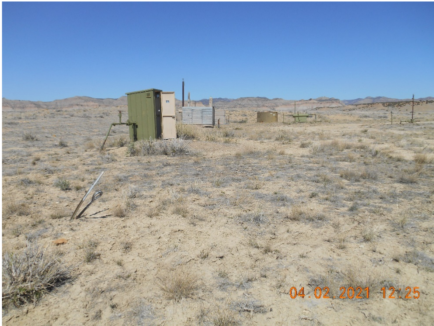
Location overview looking N.
