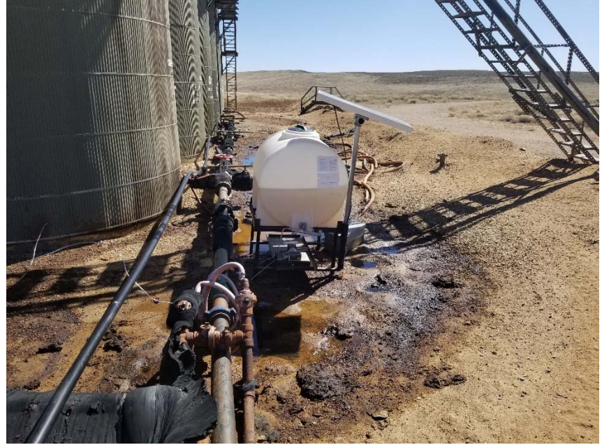
Photo 8. Spilled fluid in tank battery. Photo taken adjacent to berm breach.
