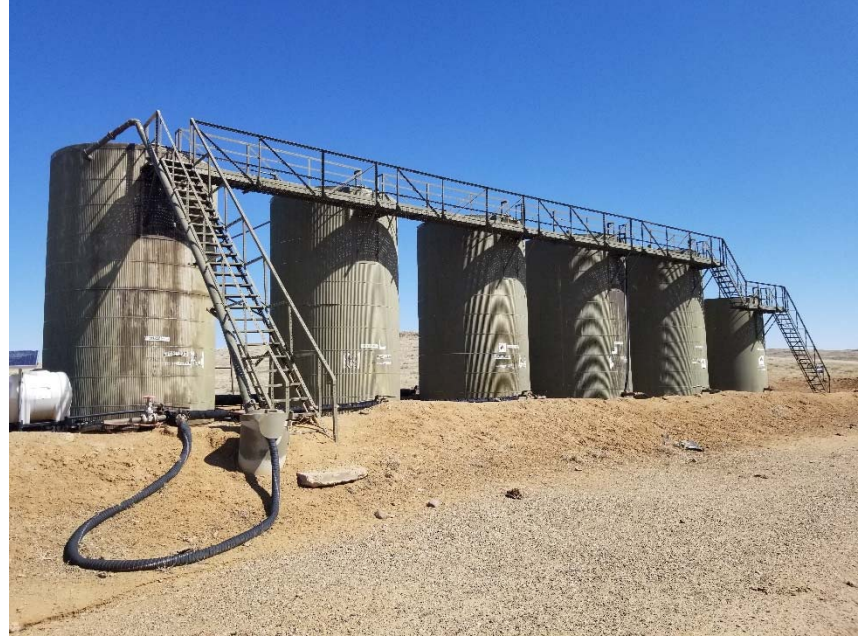
Photo 6. Tank battery with missing and incomplete tank labels.
