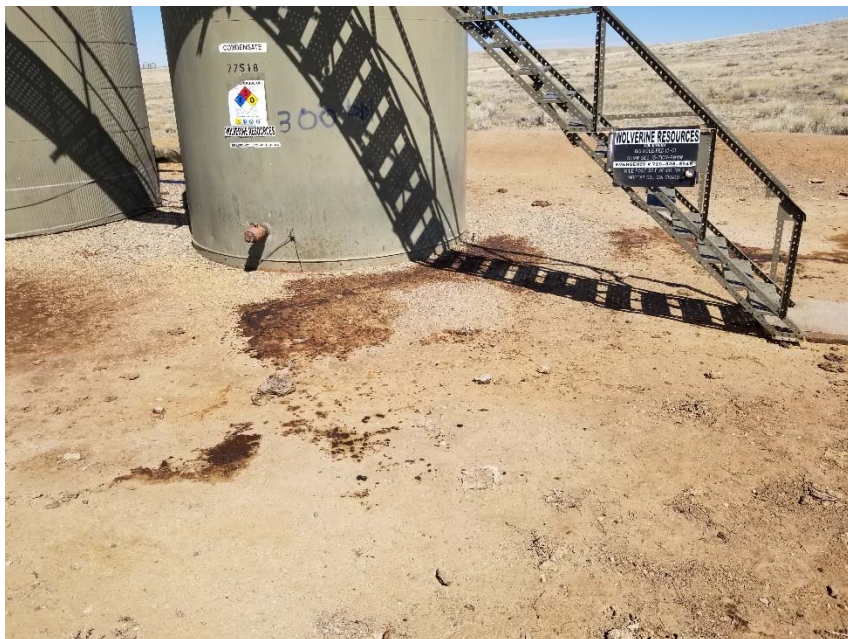
Photo 19. Stained soil in berm.
