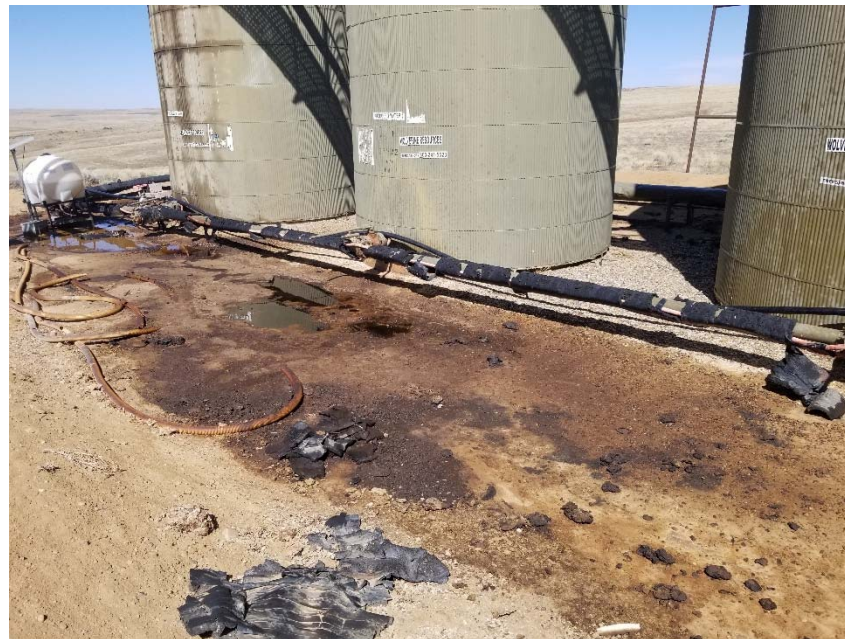
Photo 20. Stained soil in berm and fluid in berm.
