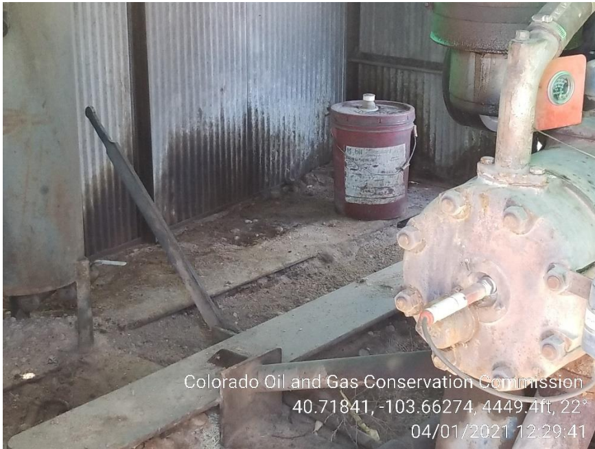
Photo 9 – Stained Soil at Gas Engine
