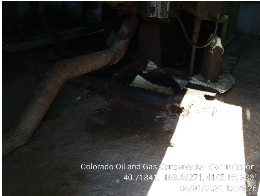
Photo 7 – Stained Soil at Gas Engine
