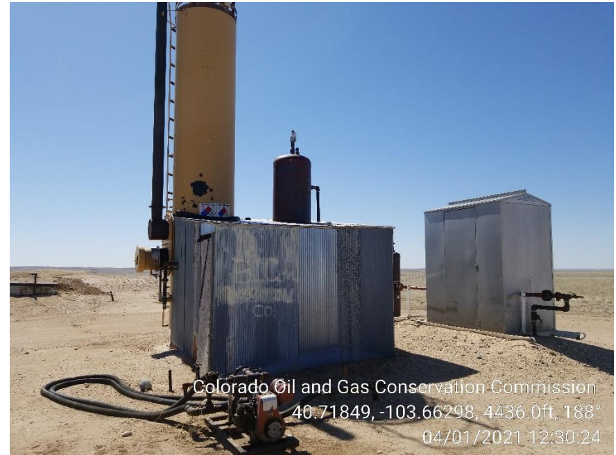
Photo 4 – Heater Treater
