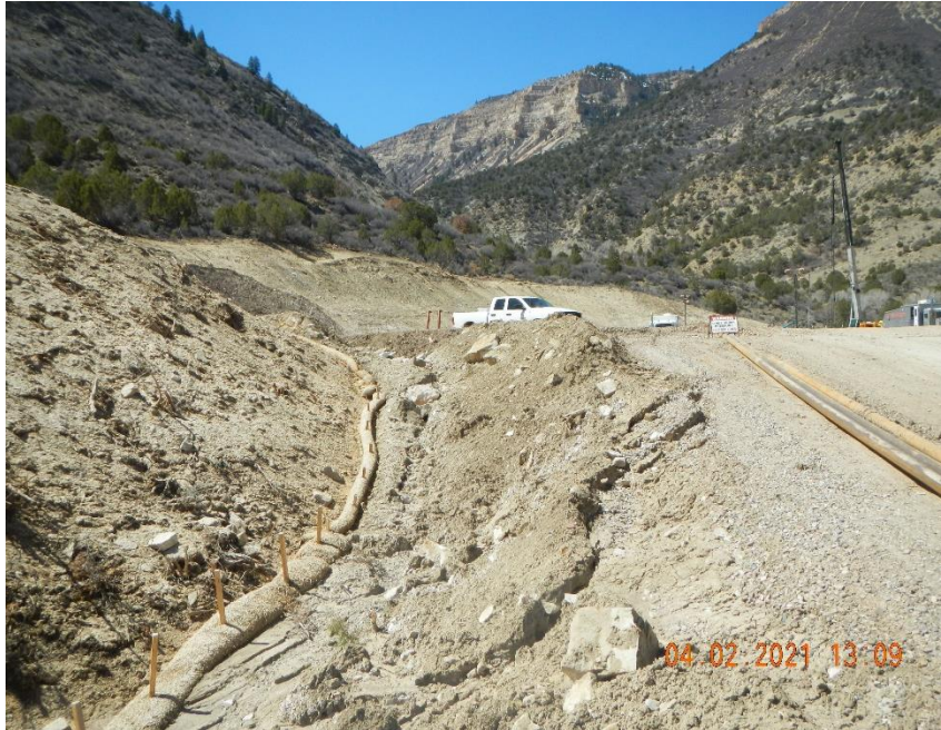
Storm water damage of ditch and shoulder of access road at entrance of location.
