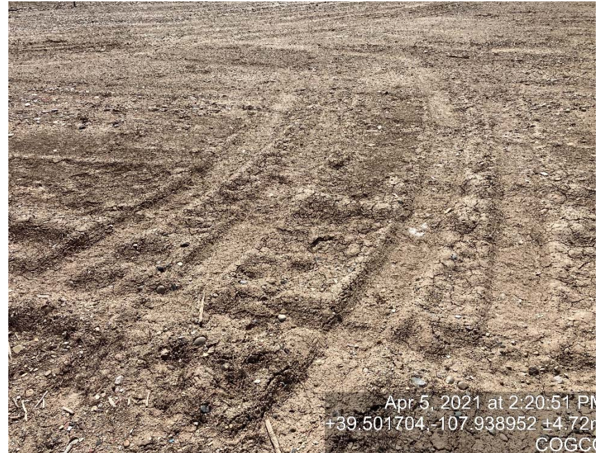
Lack of stabilization/compaction
