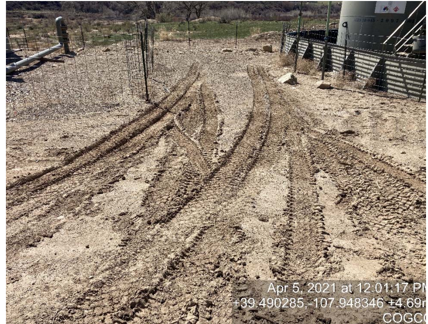
Lack of stabilization/compaction
