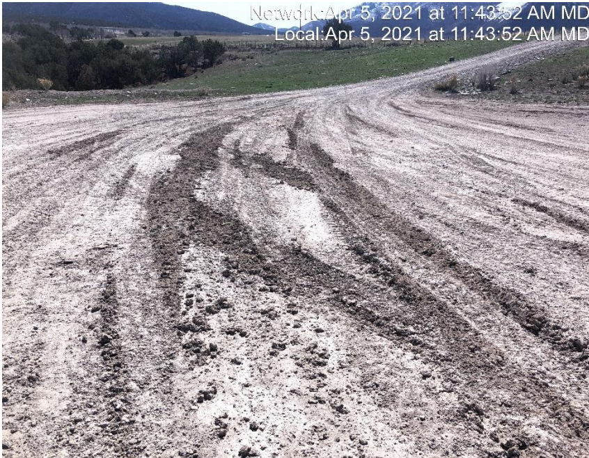
Photo #3374 No form of tracking control at entrance to location
