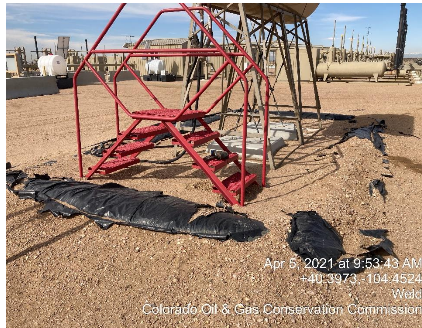
Photo #6 Inadequate Berms
