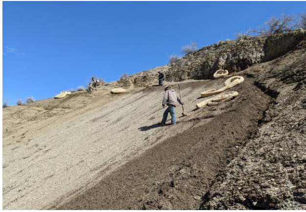
Installing Wattle above Loose Shale Material
