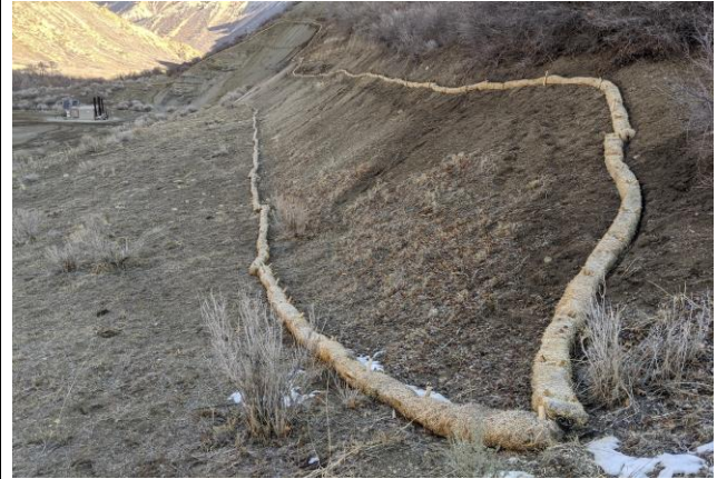
Wattle Installed on the CC 629-23-42 Pad
