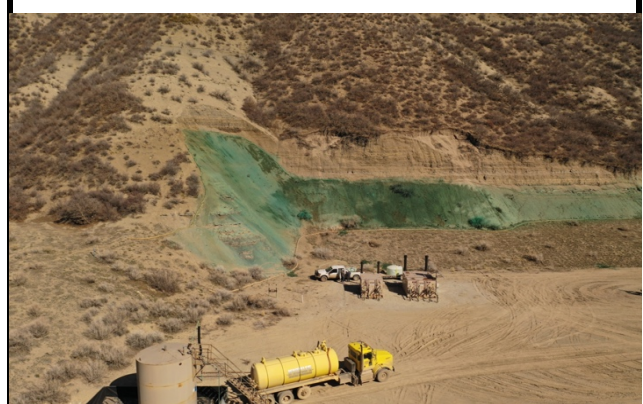
Ariel view showing the application of the hydro seeding.
