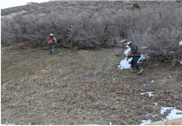
Broadcast Seeding the CC 629-23-42 Cut-Slope
