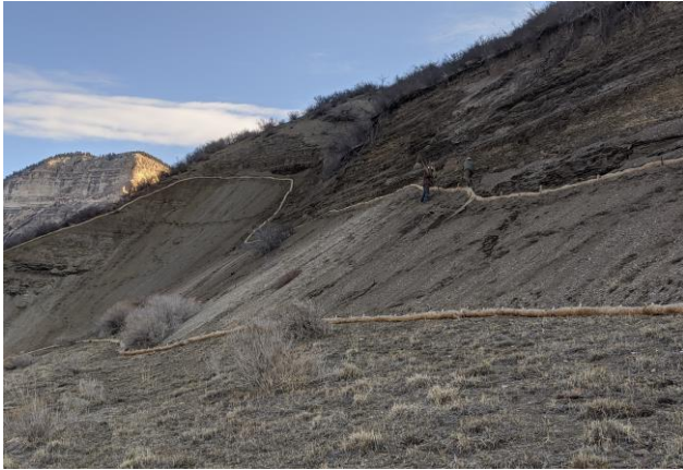
Wattle Installed on the CC 629-23-42 Pad
