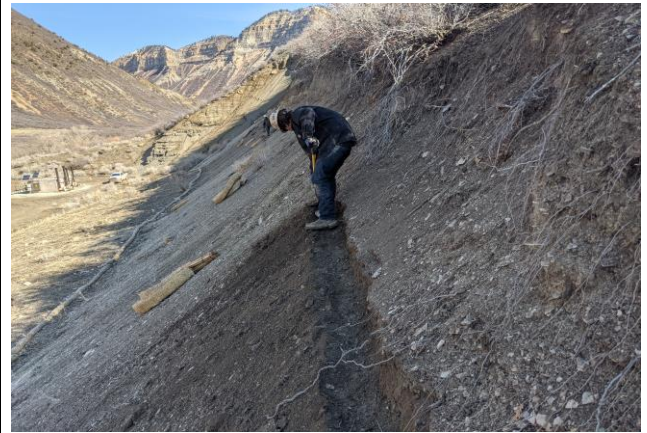
Hand Digging Trench for Wattle Installation
