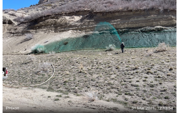
Broadcasting the hydroseed mix
