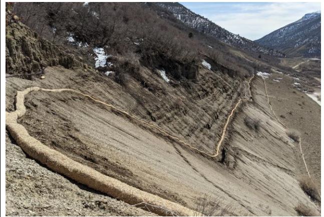
Wattle Laid Out in Preparation for Staking
