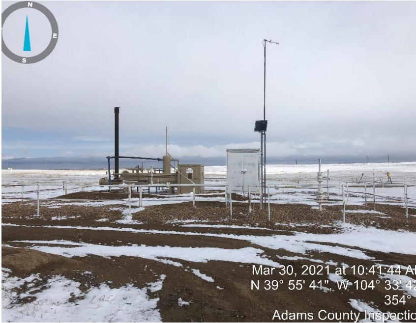
Photo #3 Separator & Meter.
