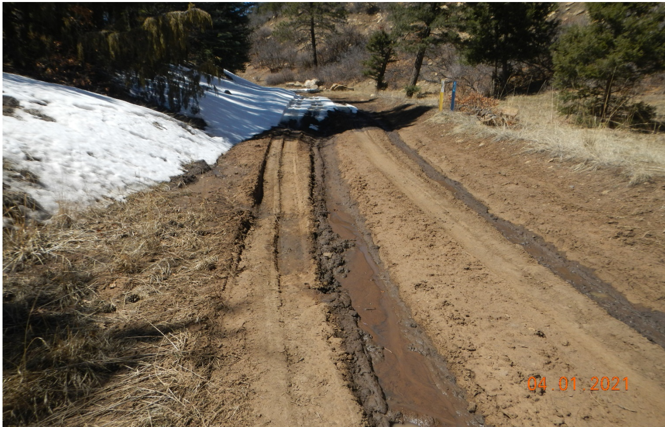
Photo 3. The road along the canyon bottom is not stabilized and maintained.
