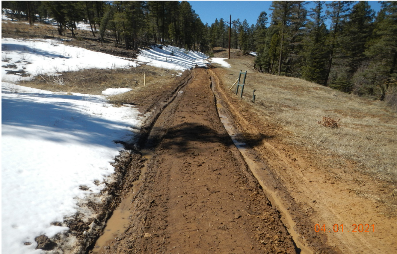
Photo 4. The road along the canyon bottom is not stabilized and maintained.
