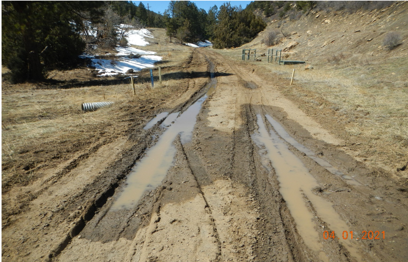
Photo 1. Facing west toward the access road at the canyon bottom near AC 1-16. The road in the canyon bottom is rutting and not maintained or stabilized.
