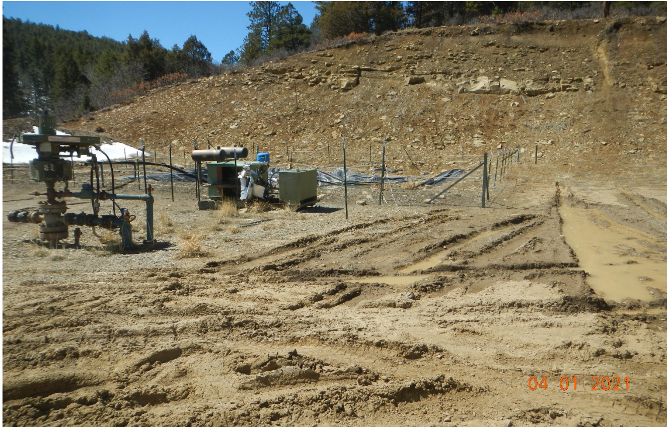
Photo 5. There is vehicle rutting on the location. The fence around the pit needs to be repaired to prevent wildlife entry.
