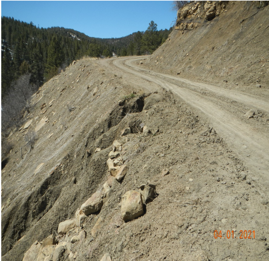
Photo 1. Facing west along the main road at Lat/Long:37.1099,-104.94878. Erosion has occurred along the fill slope of the road. This area needs to be repaired and stabilized.
