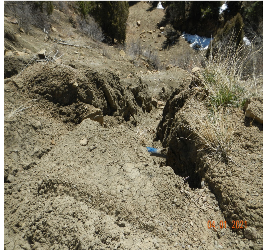
Photo 1. Facing west along the main road at Lat/Long:37.1099,-104.94878. Erosion has occurred along the fill slope of the road. This area needs to be repaired and stabilized.
