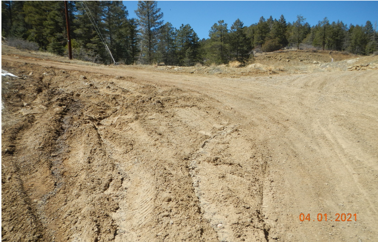
Photo 3. Facing toward the access road at right side of photo. There is rutting along the main road ascending the hill which needs to be repaired and stabilized.
