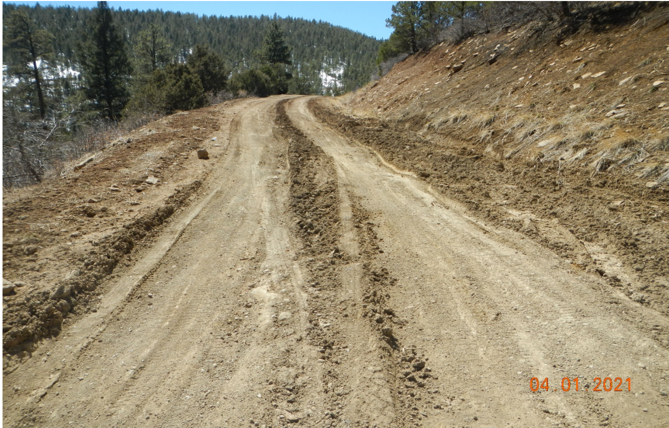
Photo 2. Facing along the main road. It appears vehicles slipped off the road causing rutting. The road needs to be repaired and stabilized.
