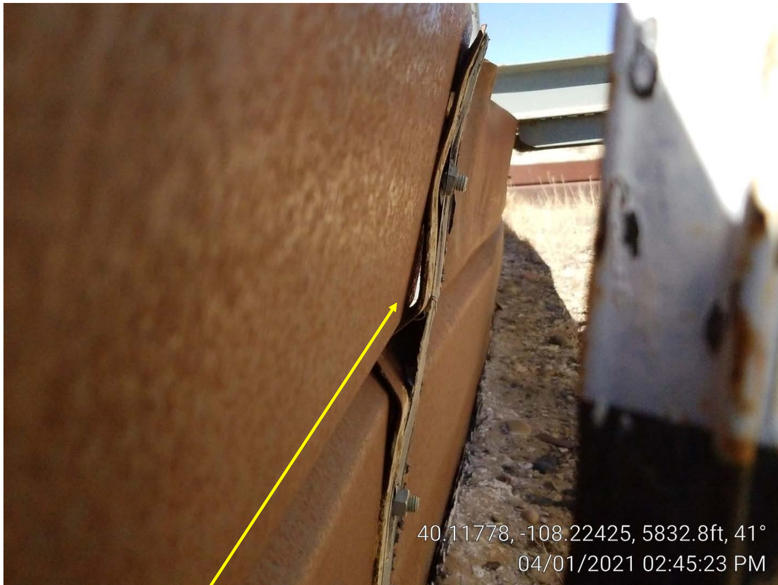
Photo 7. Gap in tank secondary containment.
