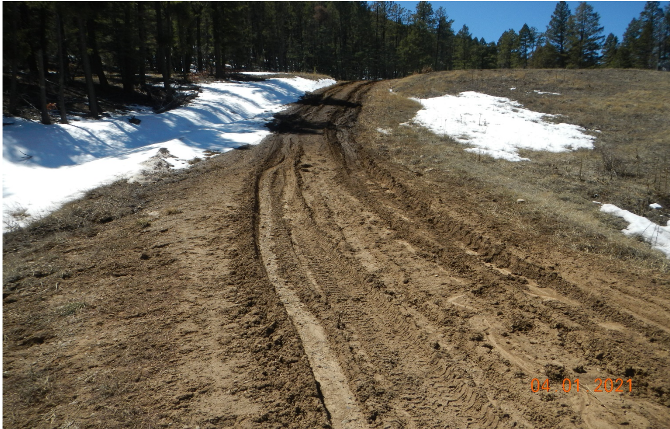
Photo 2. Facing toward the access road. The access road is rutted and not stabilized and maintained.
