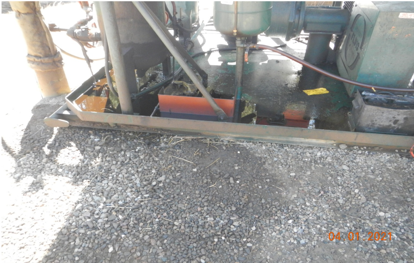
Photo 5. There is oil stained soil and oil in the engine skid which needs to be cleaned up.
