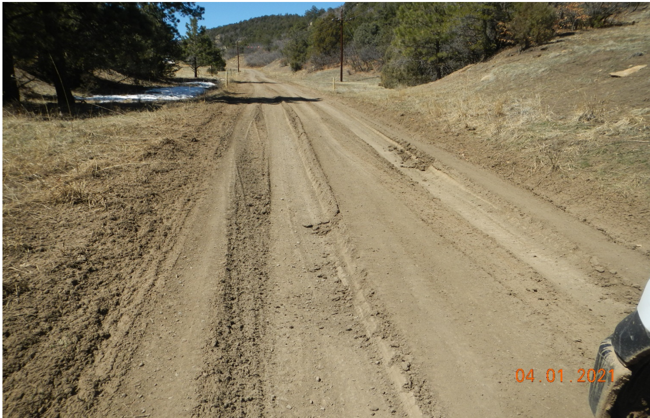
Photo 1. There are areas along the main road which are rutted and not maintained.
