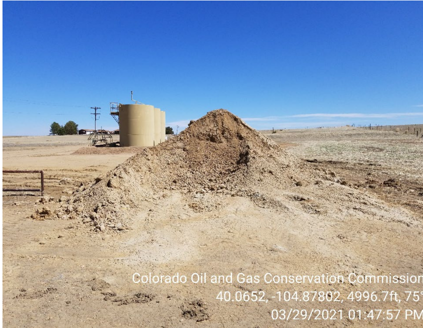
Photo 3 – Soil stockpiled on site with no BMPs
