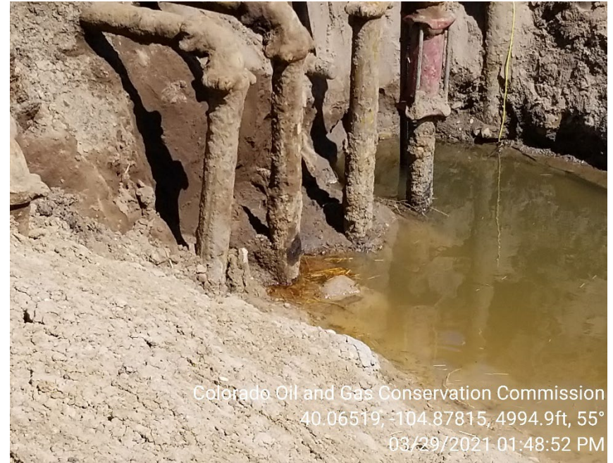
Photo 2 – Impacted soils appear to still be in place in excavation wall adjacent to header. Hydrocarbon sheen visible on groundwater in excavation.
