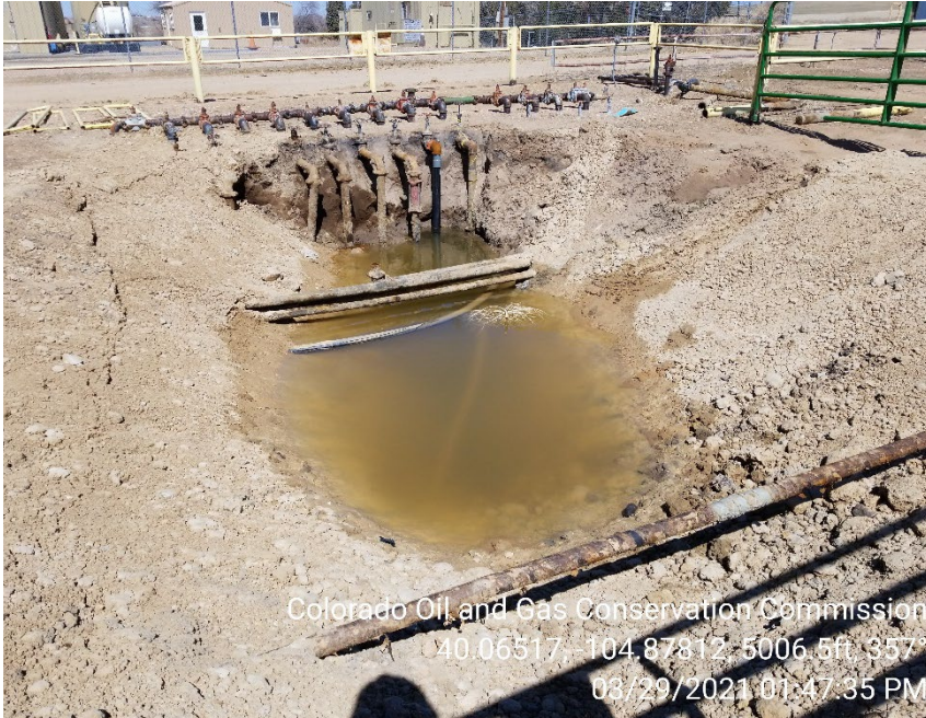
Photo 1 – Open spill excavation; impacted soils appear to still be in place in excavation wall adjacent to header. Hydrocarbon sheen visible on groundwater in excavation.
