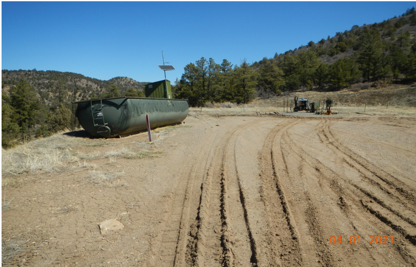
Photo 2. Facing toward the location. There is no secondary containment around the PW tank.
