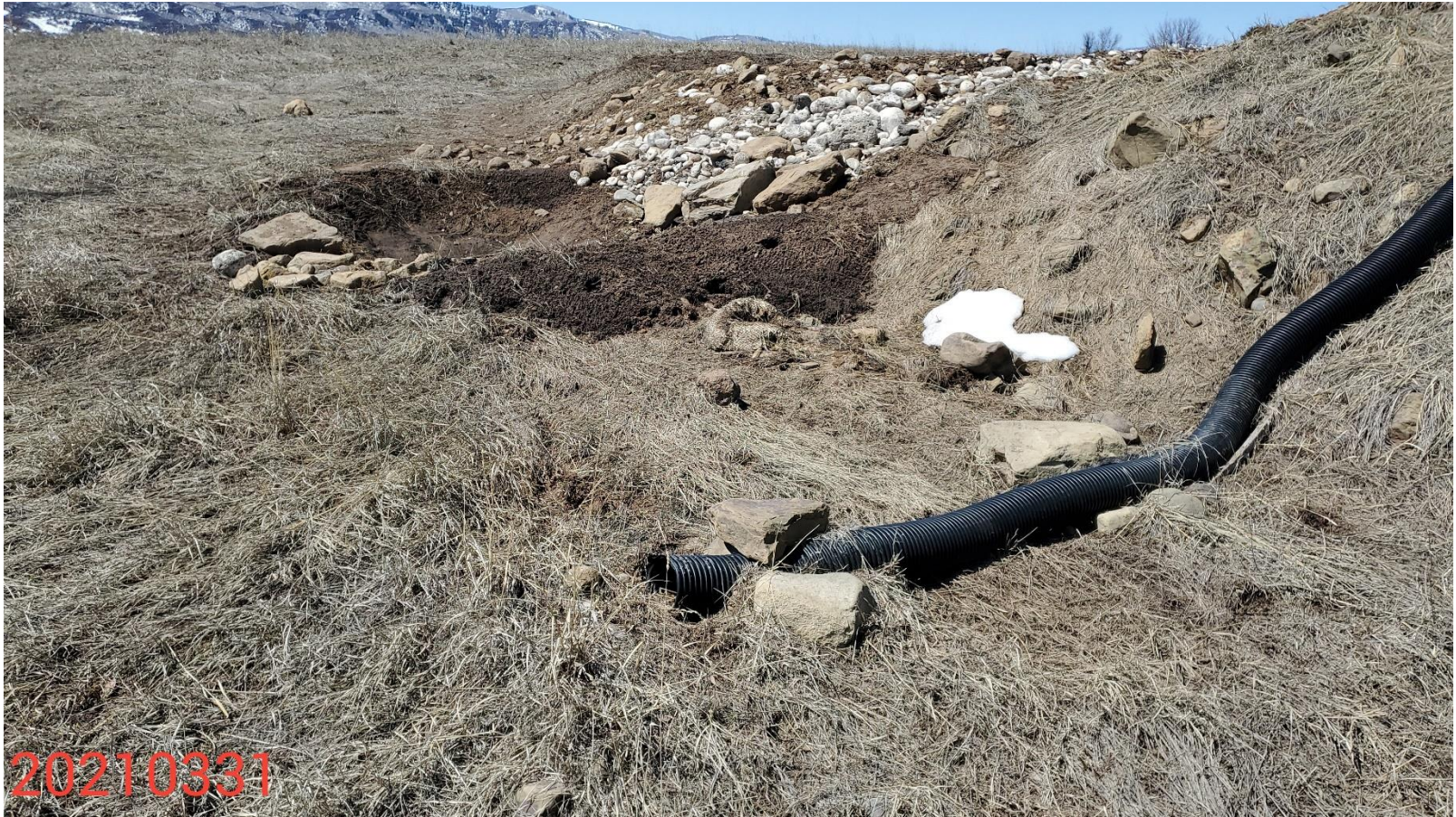
Photo 4: Photo taken from the southwest end of the Location. Photo shows slope drain outlet, sediment trap and ditch; BMPs have not been installed in accordance with good engineering practices.
