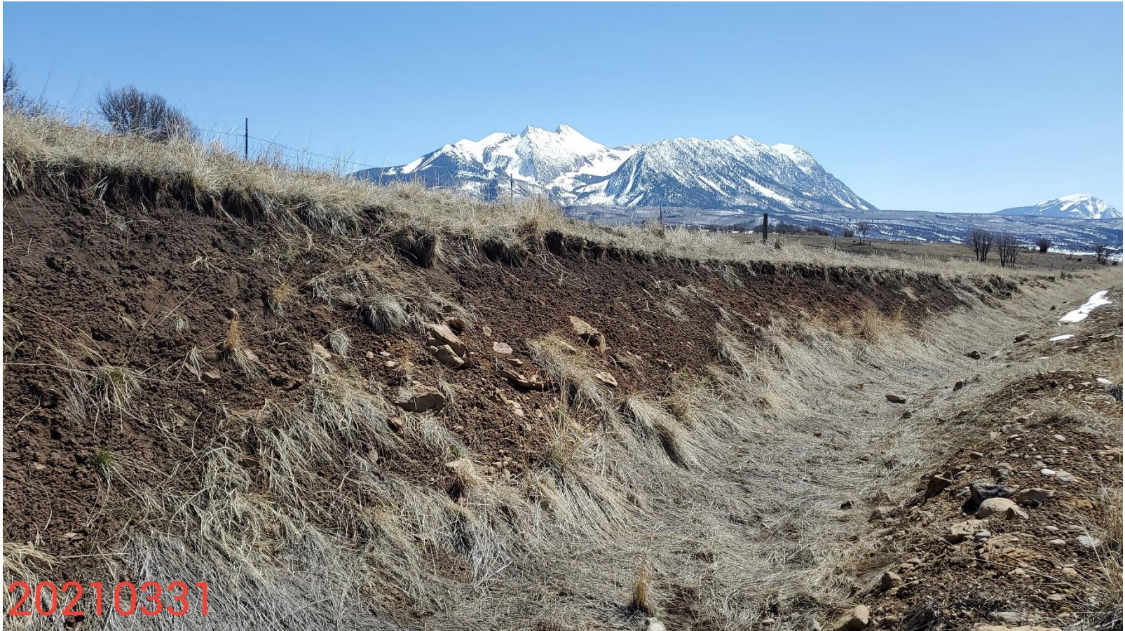
Photo 12: Photo taken from the cut slopes on the northeast end of the Location. Photo shows control measures to stabilize and protect slopes on the Location remain missing or insufficient.
