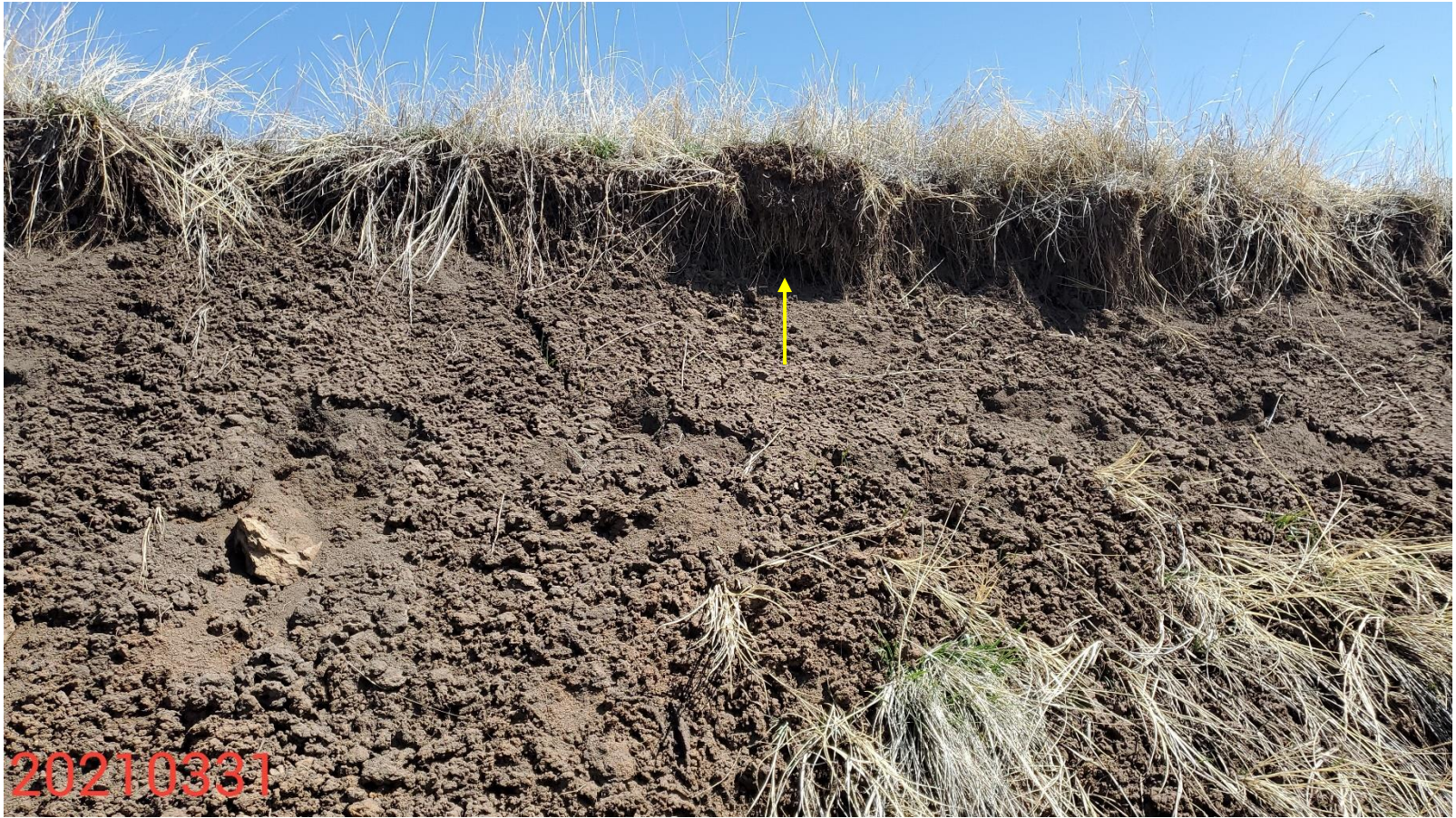
Photo 13: Photo taken from the cut slopes on the northeast end of the Location. Photo shows control measures to stabilize and protect slopes on the Location remain missing or insufficient. Photo also shows example of erosion that has cut beneath vegetation and plant roots, compromising stability.
