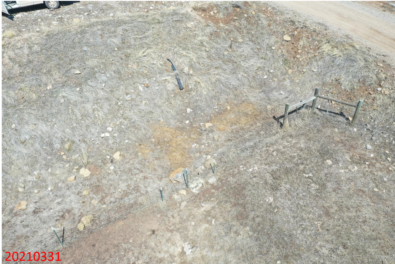
Photo 3: Aerial image showing slope drain on the southeastern end of the Location; Slope drain has not been constructed with an appropriate outlet per good engineering practices
