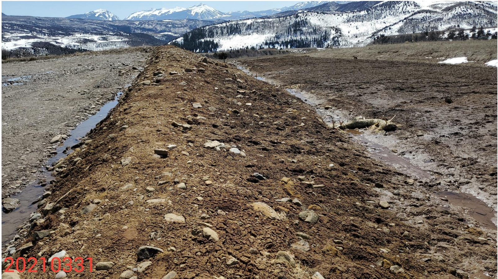
Photo 8: Photo taken from the slopes on the west end of the Location, facing south. Photo shows control measures to stabilize and protect slopes on the Location remain missing or insufficient.
