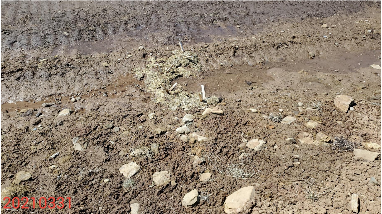
Photo 9: Photo taken from the west end of the Location. Photo shows example of wattle control measures implemented as velocity checks that have not been maintained in a proper functioning condition.
