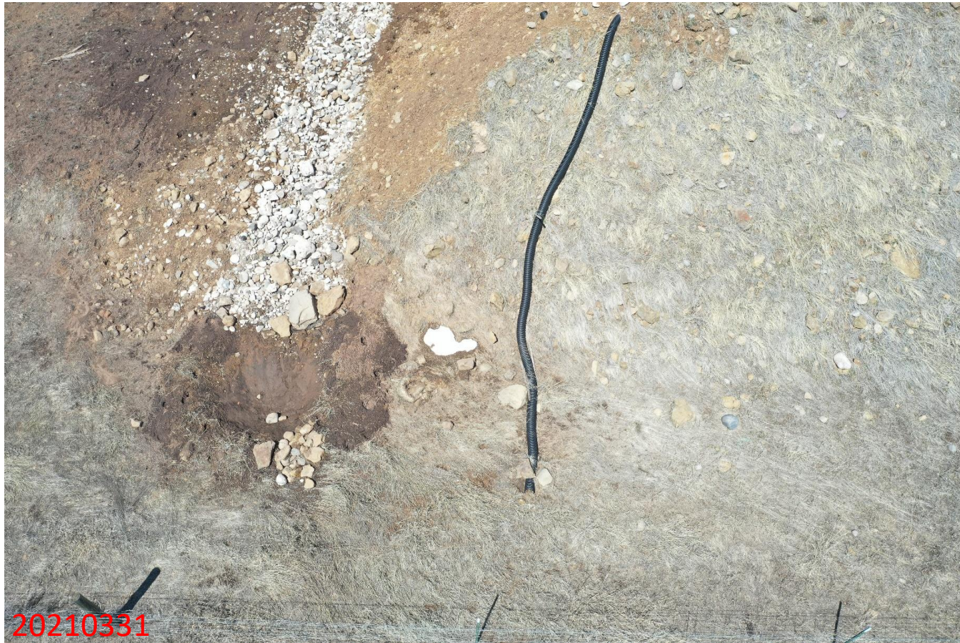
Photo 2: Aerial image showing sediment trap, ditch and slope drain on the southwestern end of the Location; Slope drain has not been constructed with an appropriate outlet per good engineering practices.
