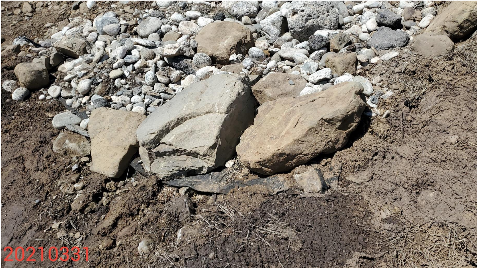
Photo 5: Photo shows stormwater ditch; inlet to sediment trap has been lined and armored with various sized aggregate, however, rounded river stone appears to have been utilized in the ditch, and is not considered a good engineering practice.
