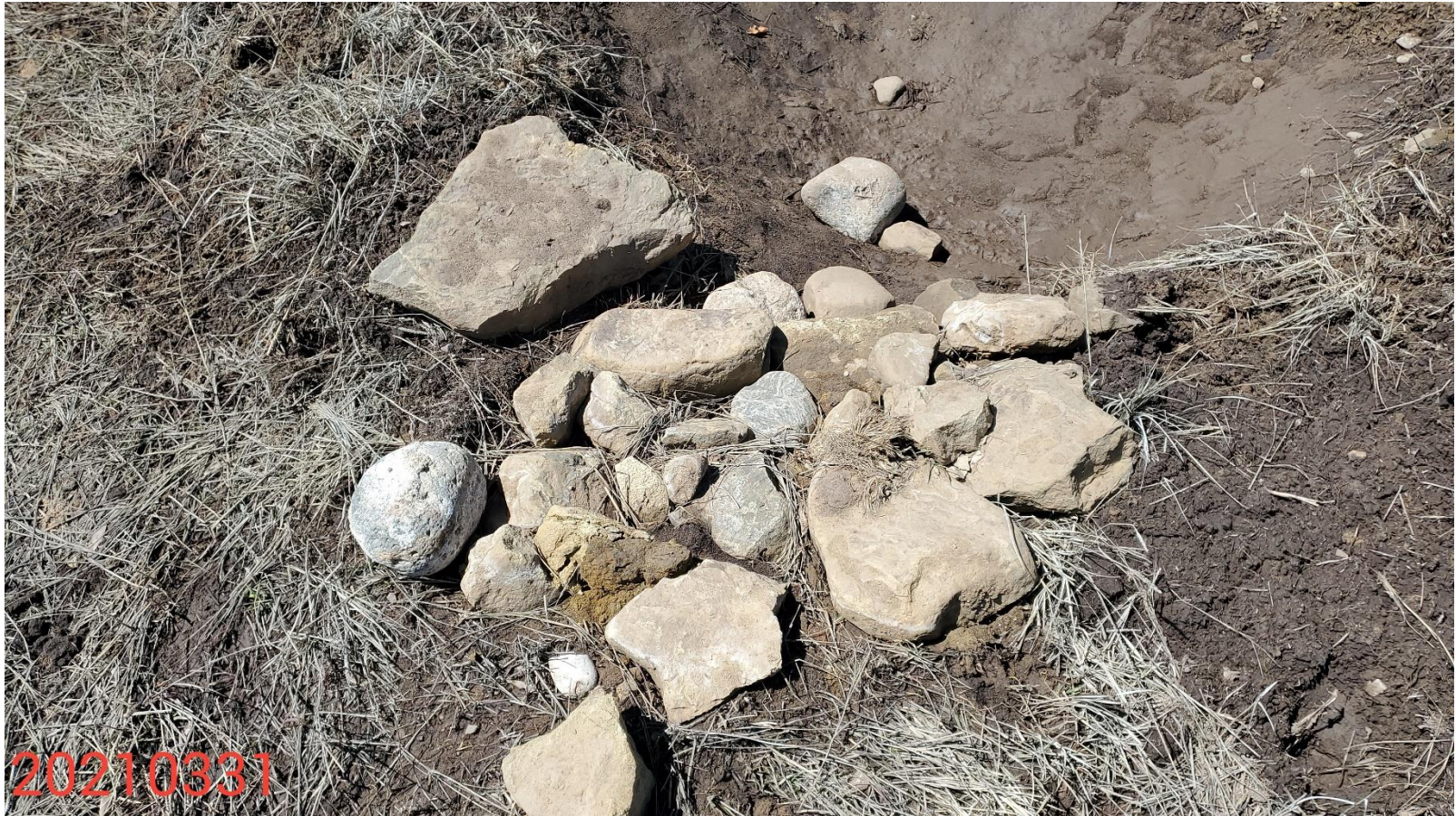
Photo 6: Photo taken from the northeast corner of the Location. Photo shows outlet at sediment trap; BMP has not been constructed in accordance with good engineering practices.
