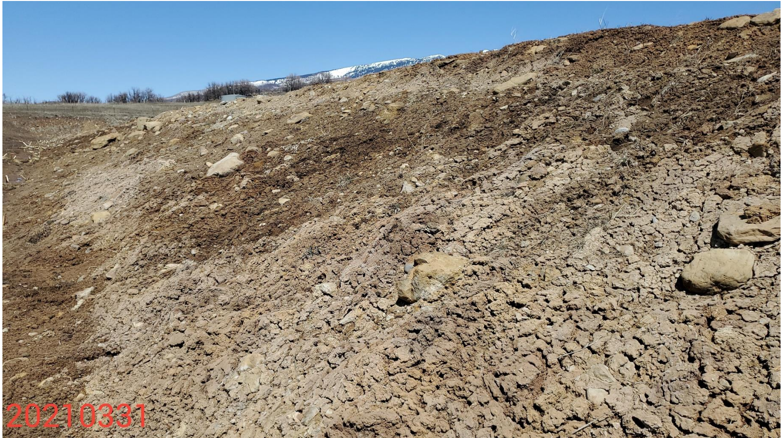
Photo 7: Photo taken from the slopes on the west end of the Location, facing north. Photo shows control measures to stabilize and protect slopes on the Location remain missing or insufficient.
