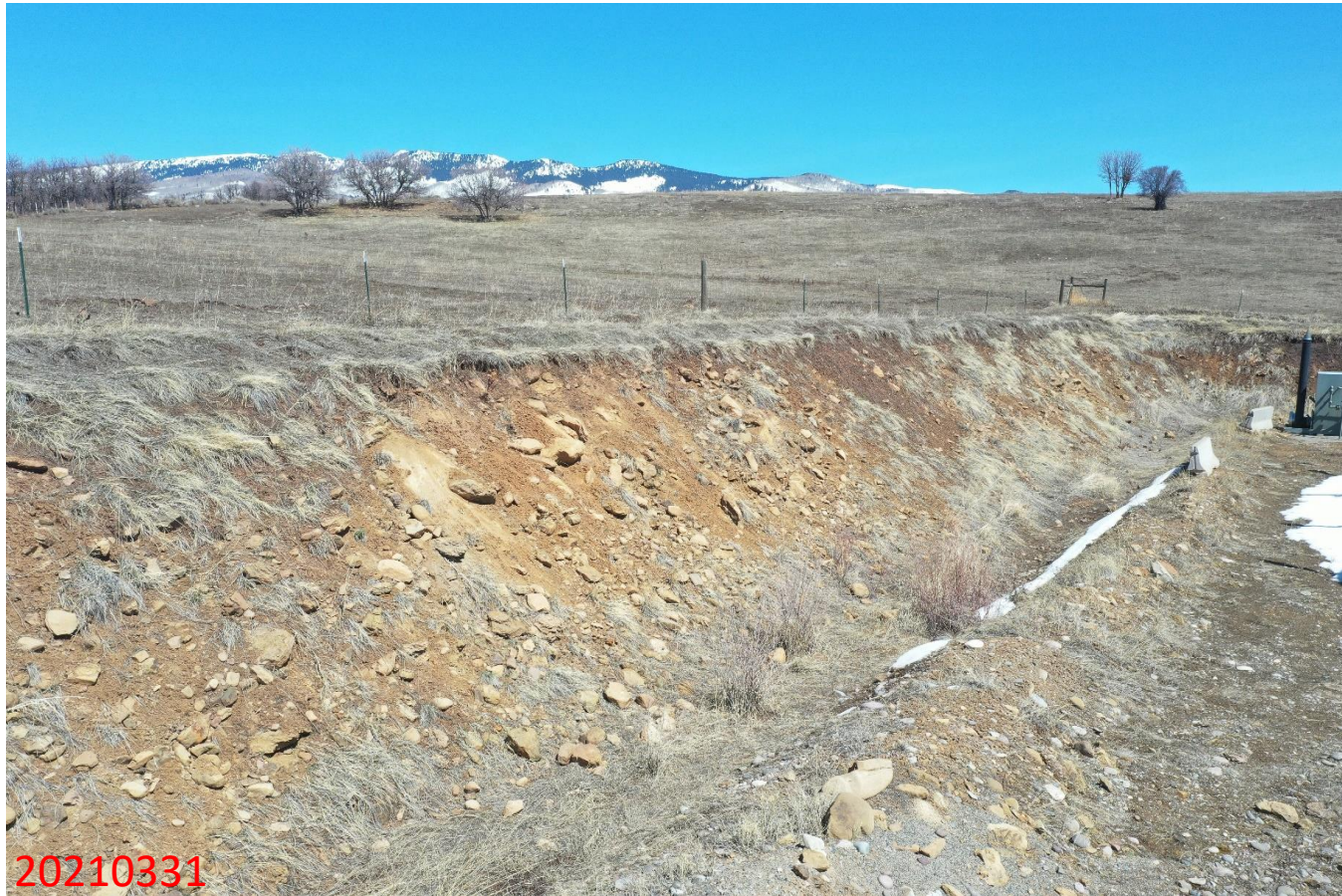
Photo 10: Photo taken from the cut slopes on the north end of the Location. Photo shows control measures to stabilize and protect slopes on the Location remain missing or insufficient.
