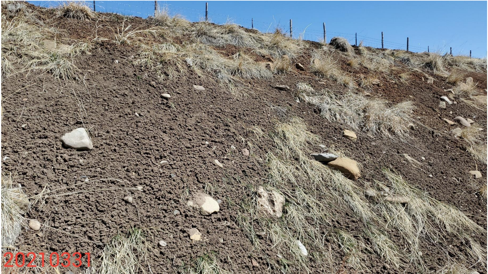
Photo 6: Photo taken from the cut slopes of the Location. Photo shows control measures to stabilize/protect slopes on the Location remain missing or insufficient in accordance with Rule 1002.f.(2)C.
