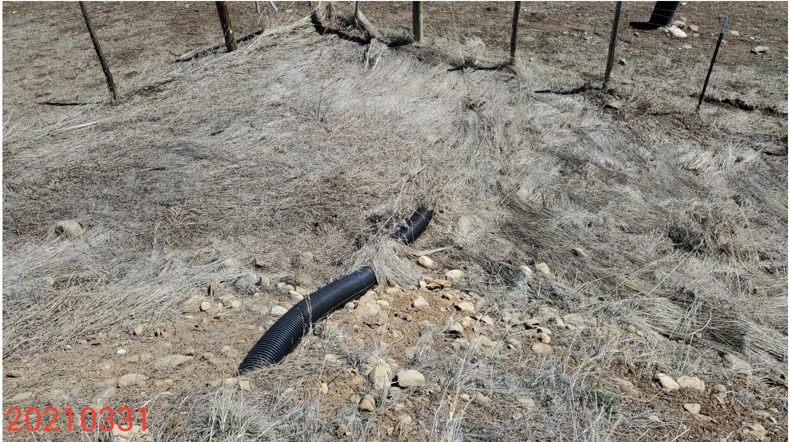
Photo 8: Photo taken from the northeast corner of the Location. Photo shows example of slope drain that has not been constructed with an appropriate outlet in accordance with good engineering practices.
