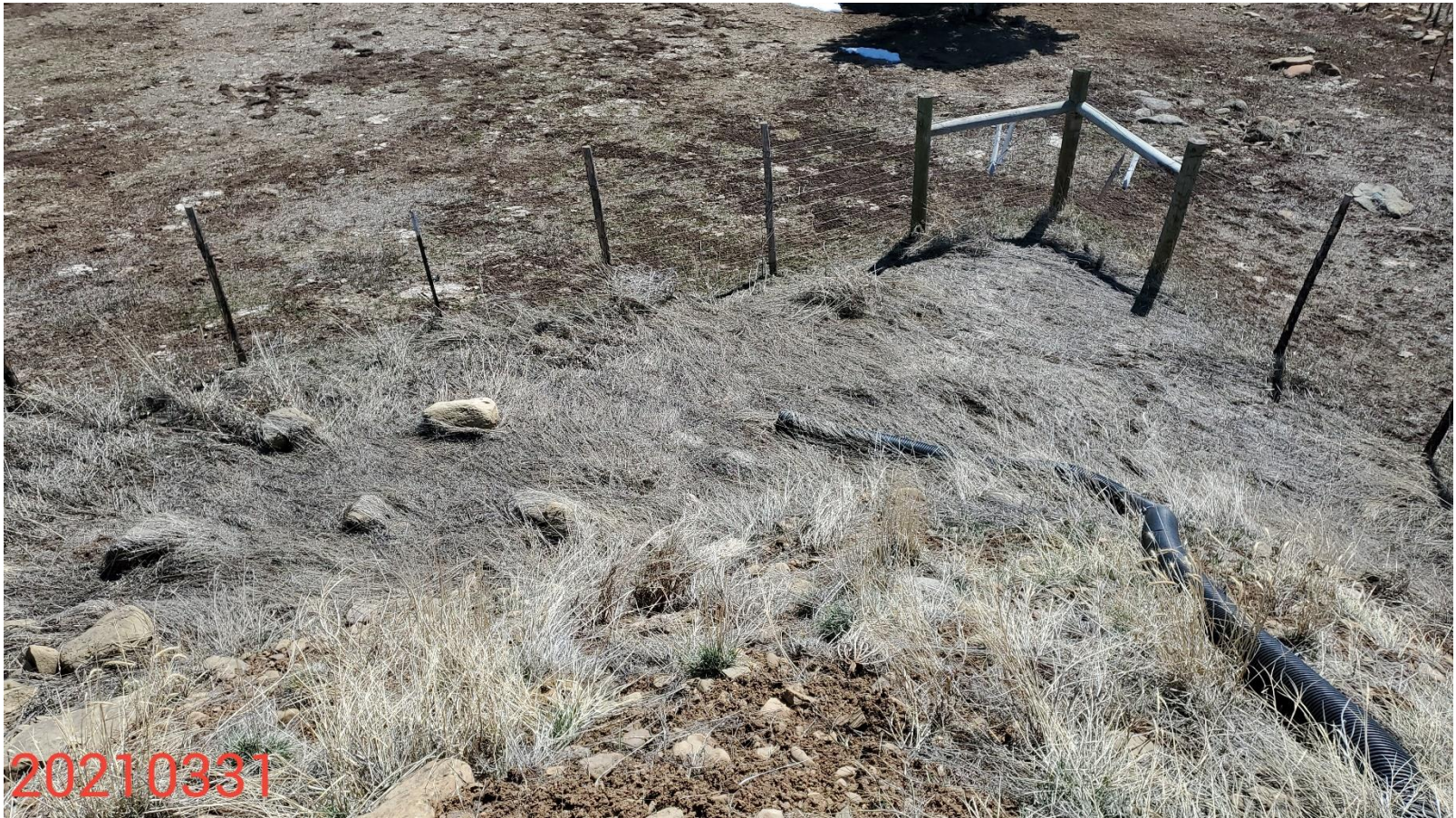
Photo 7: Photo taken from the southeast corner of the Location. Photo shows example of slope drain that has not been constructed with an appropriate outlet in accordance with good engineering practices.
