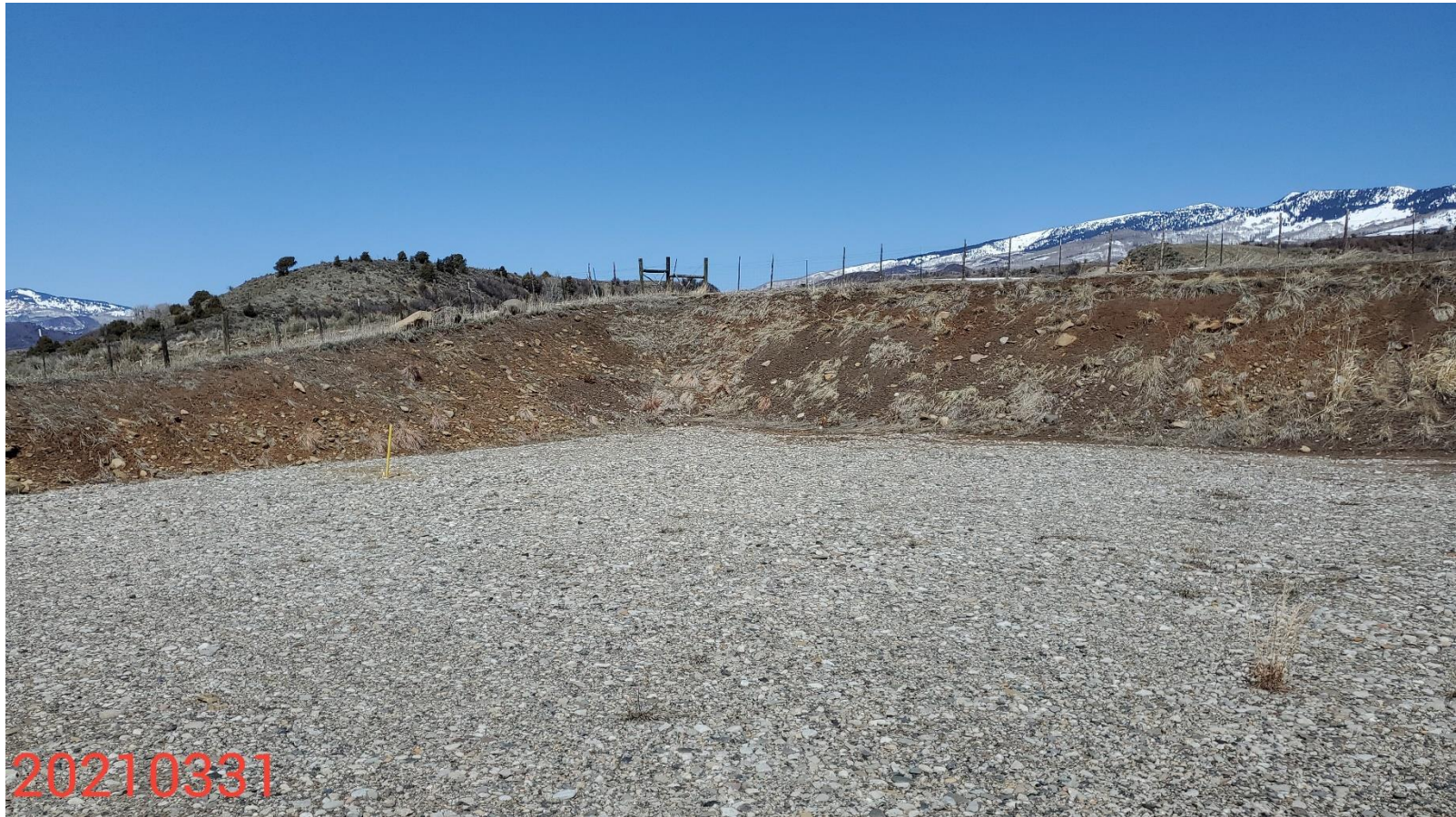
Photo 4: Photo taken from the Location, facing northwest. Photo shows cut slopes of the Location. Previous inspection required Operator to implement control measures to stabilize/protect slopes of the Location; BMPs remain missing or insufficient to stabilize/protect slopes of the Location in accordance with Rule 1002.f.(2)C.
