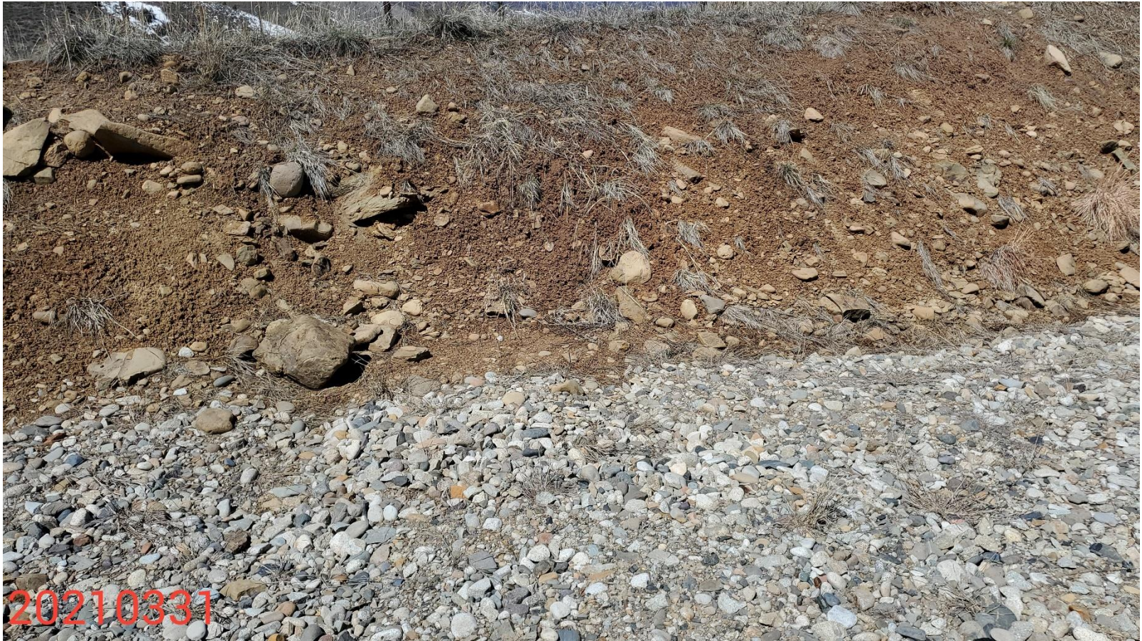
Photo 5: Photo taken from the cut slopes of the Location. Photo shows control measures to stabilize/protect slopes on the Location remain missing or insufficient in accordance with Rule 1002.f.(2)C.
