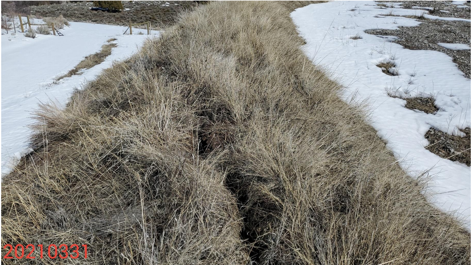
Photo 2: Photo taken from the top of the berm along the northern perimeter of the Pad. Photo shows example of crack/stabilization issues observed throughout the perimeter of the Location and slopes.
