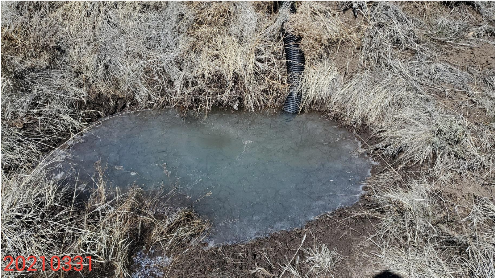
Photo 5: Photo taken from the south end of the Location. Photo shows Sediment trap has not been constructed in accordance with good engineering practices; BMP not constructed with an appropriate inlet/outlet.
