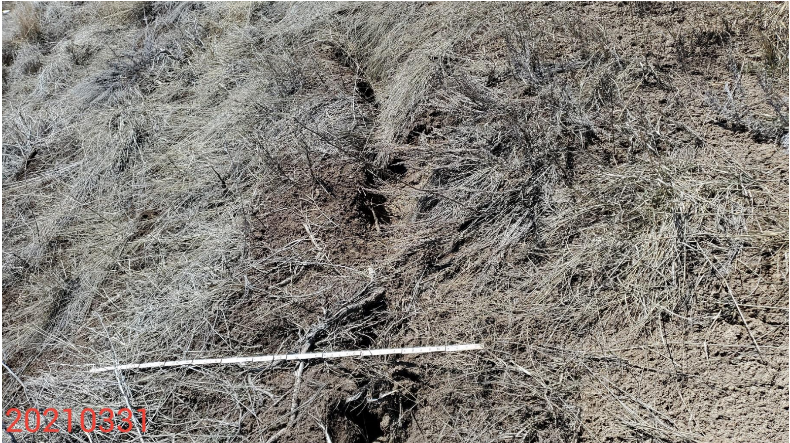
Photo 3: Photo taken from the slopes on the southeast end of the Location. Photo shows example of crack/stabilization issues observed throughout the perimeter of the Location and slopes. 6 foot measuring stick for reference.
