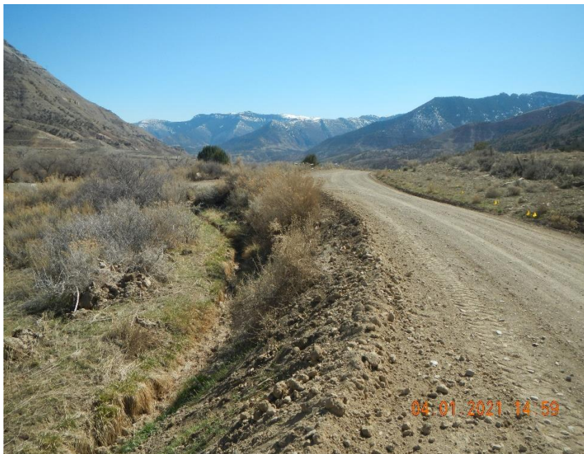
Sediment being bladed off shoulder of road.
