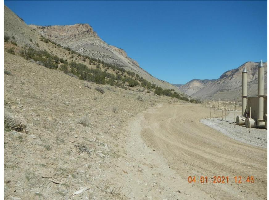
**Perimeter ditch needs cleaned out.**
