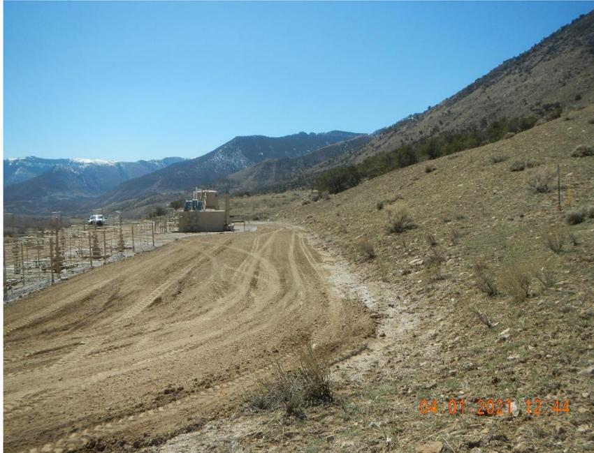
**Perimeter ditch needs cleaned out.**
