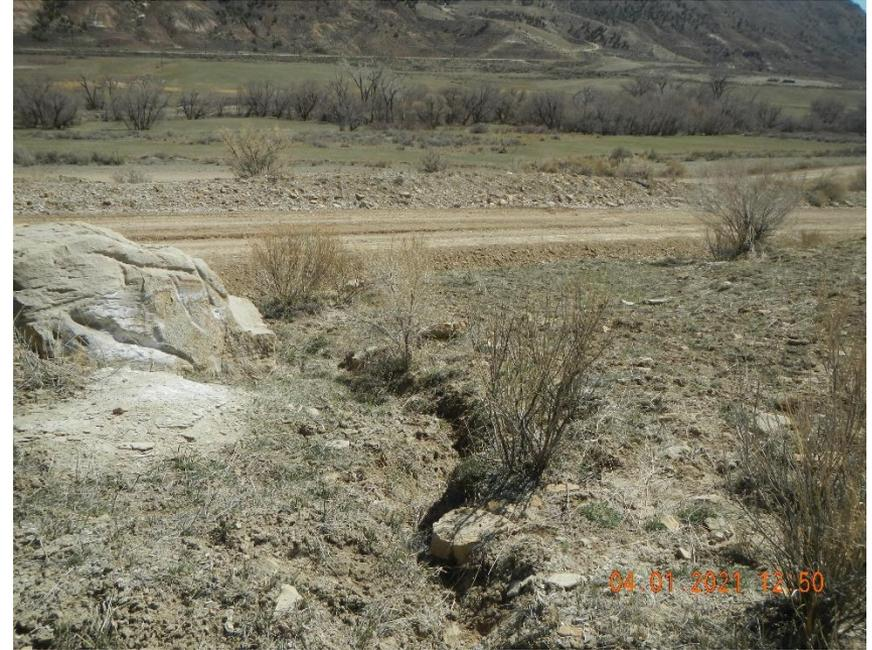
**Erosion from the storm water flow coming from check dam.**
