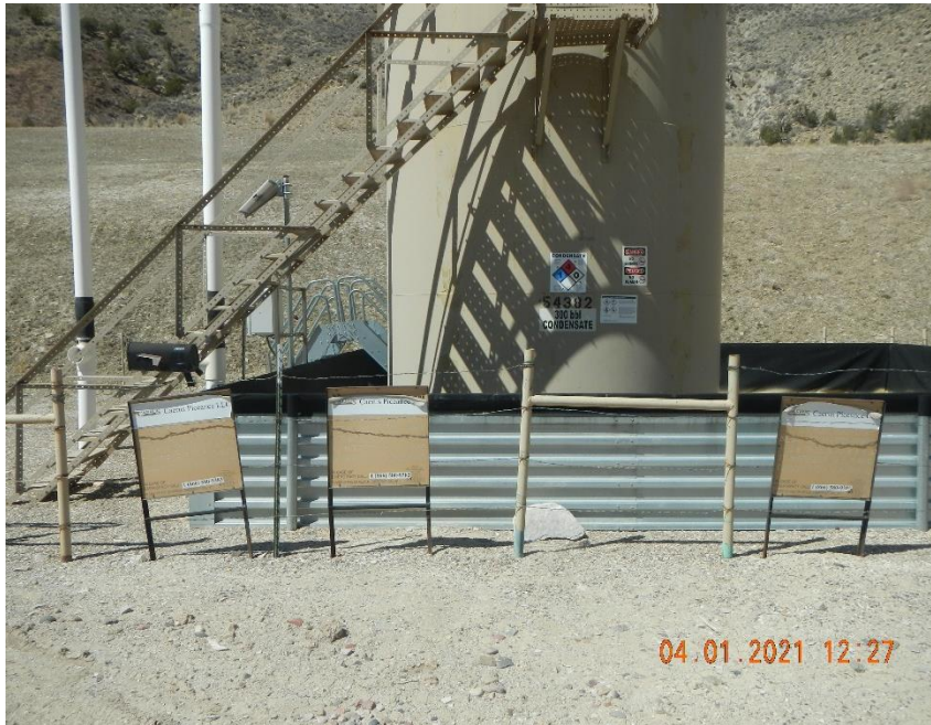
Battery signs lack contrast to be seen from distance.
