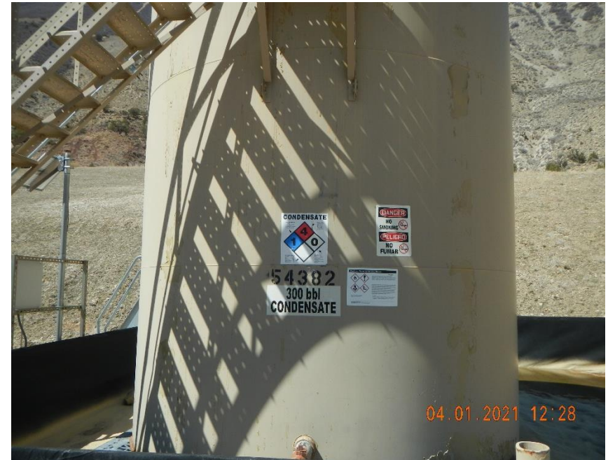
Operator name and number not on tank.
