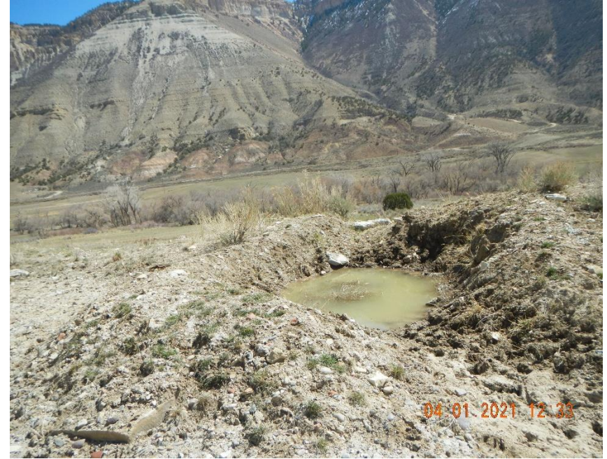
Check dam with rip rap over flow.
