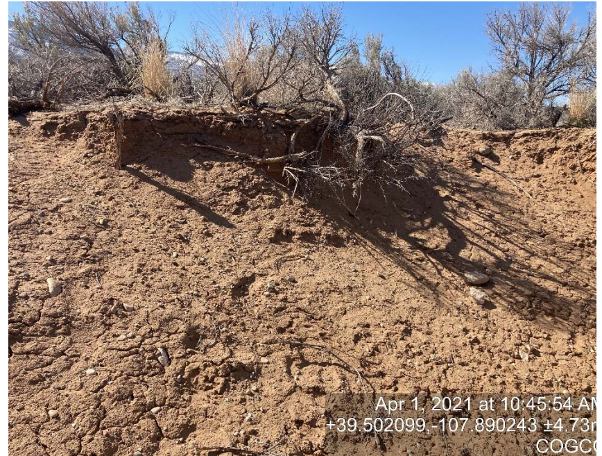
Lack of stabilization on cut slope
