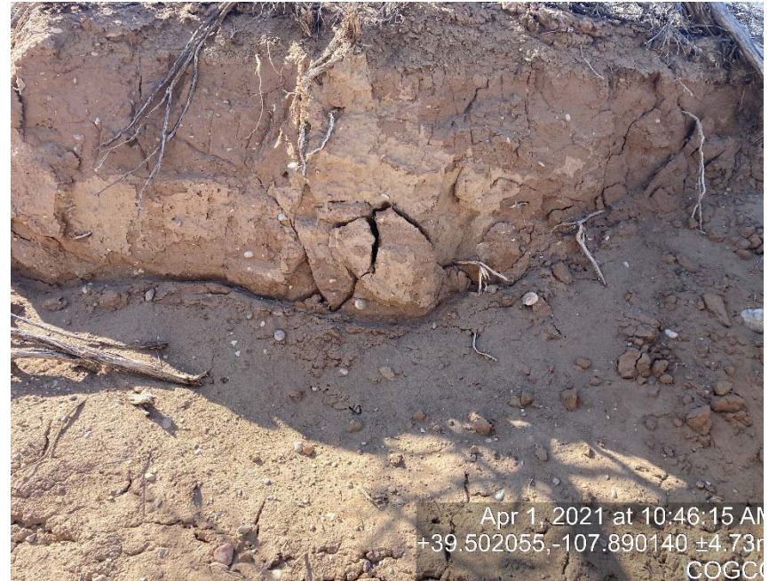
Lack of stabilization on cut slope
