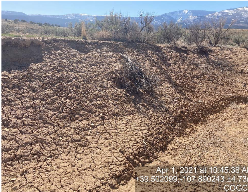
Lack of stabilization on cut slope
