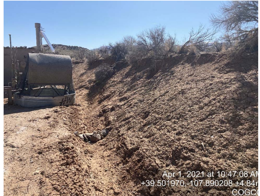
Lack of stabilization on cut slope
