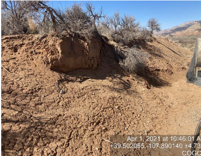
Lack of stabilization on cut slope
