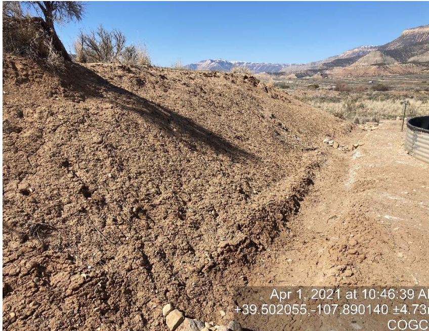
Lack of stabilization on cut slope
