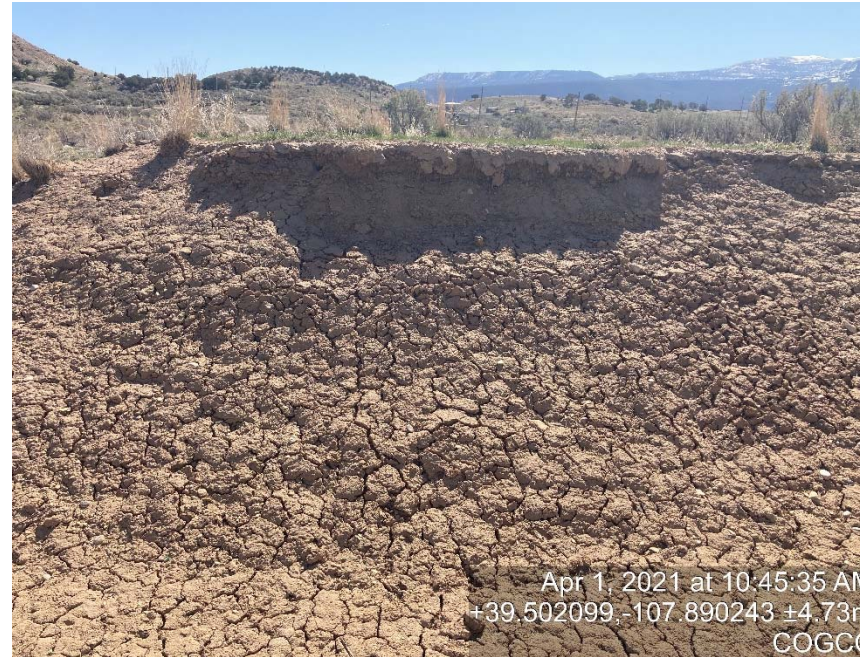
Lack of stabilization on cut slope
