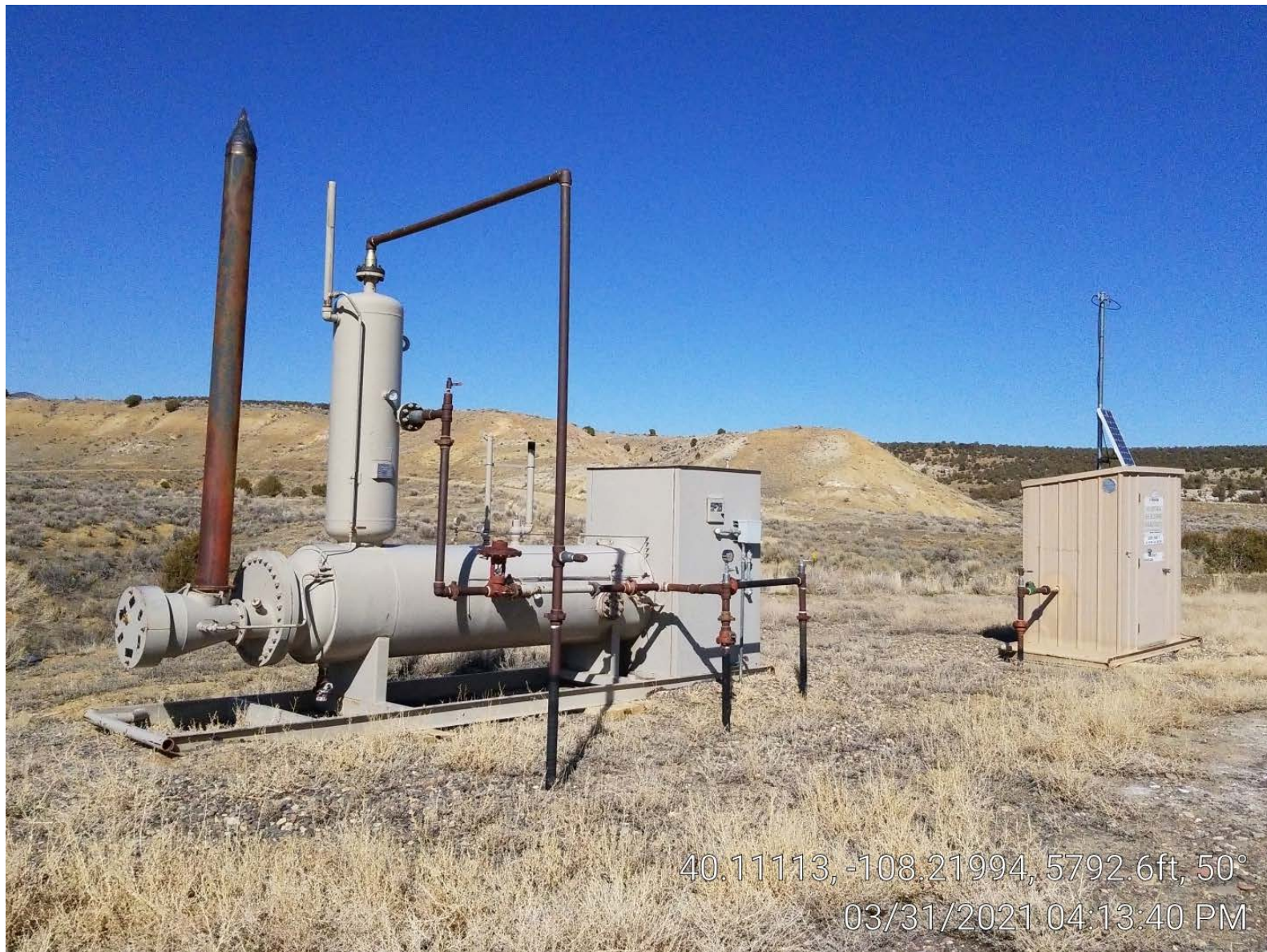
Photo 3. Separator & meter building.
