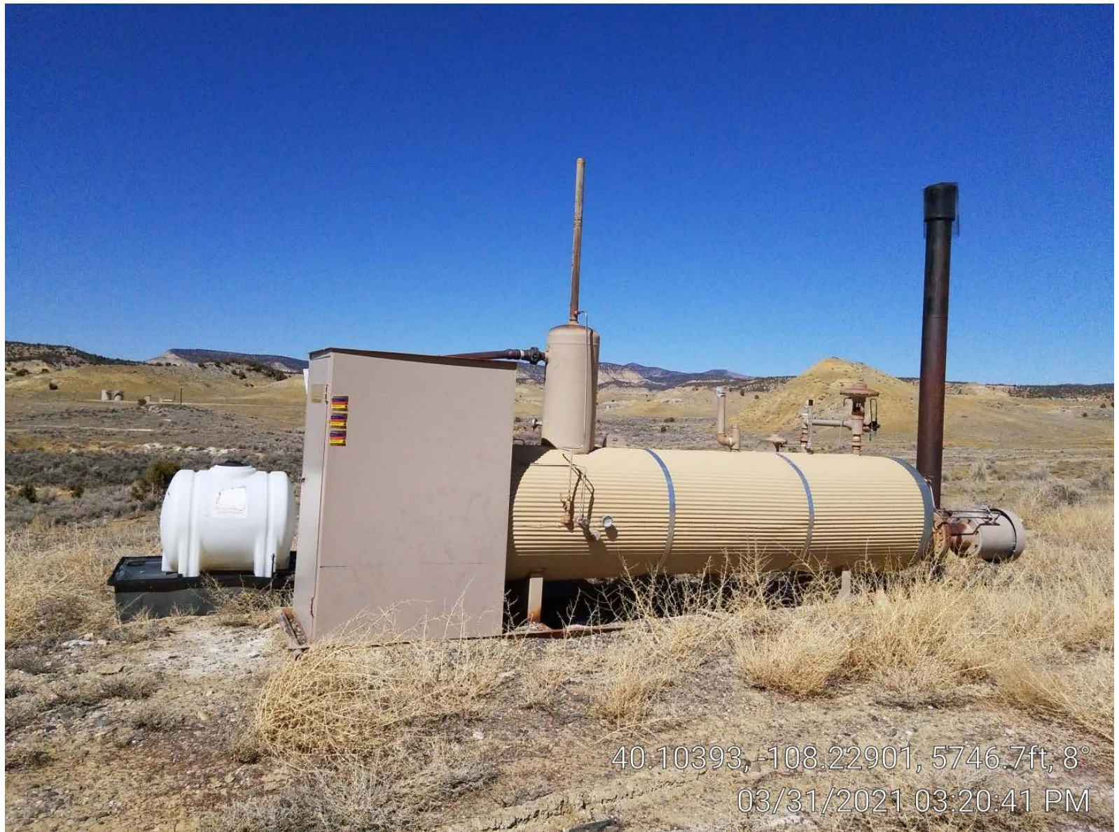
Photo 4. Horizontal separator.
