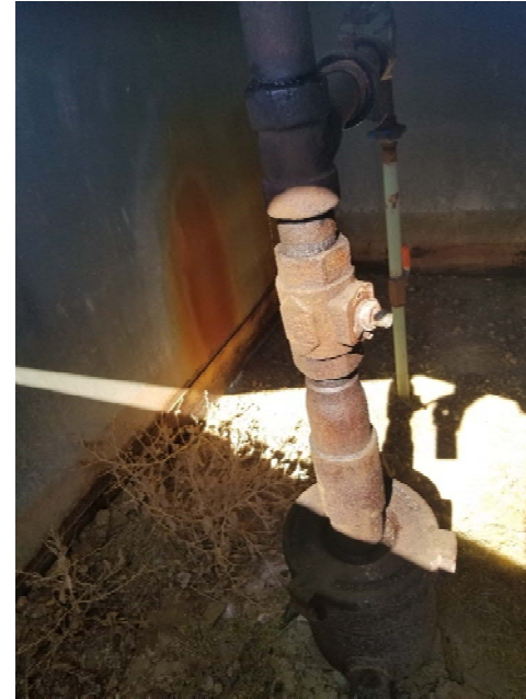
Photo 2. No bradenhead access apparent.
