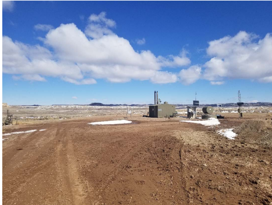
Photo 1. Overview of location taken facing north.
