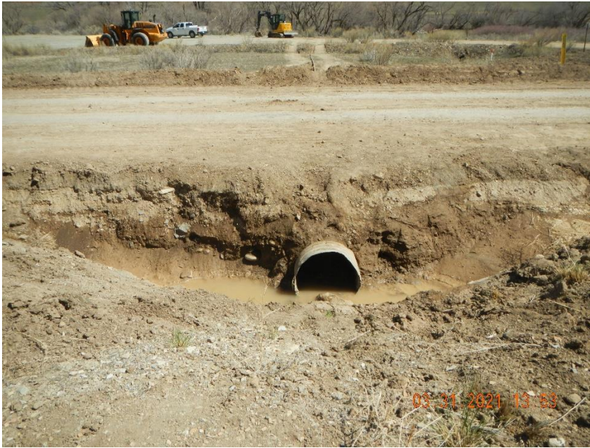
Crew working to clean out culvert.
