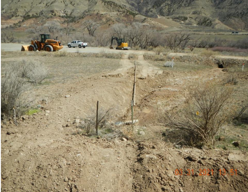
Culvert in process of being cleaned out.
