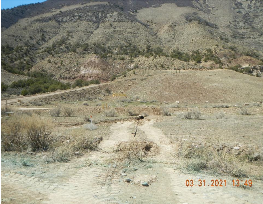
Culvert in process of being cleaned out.
