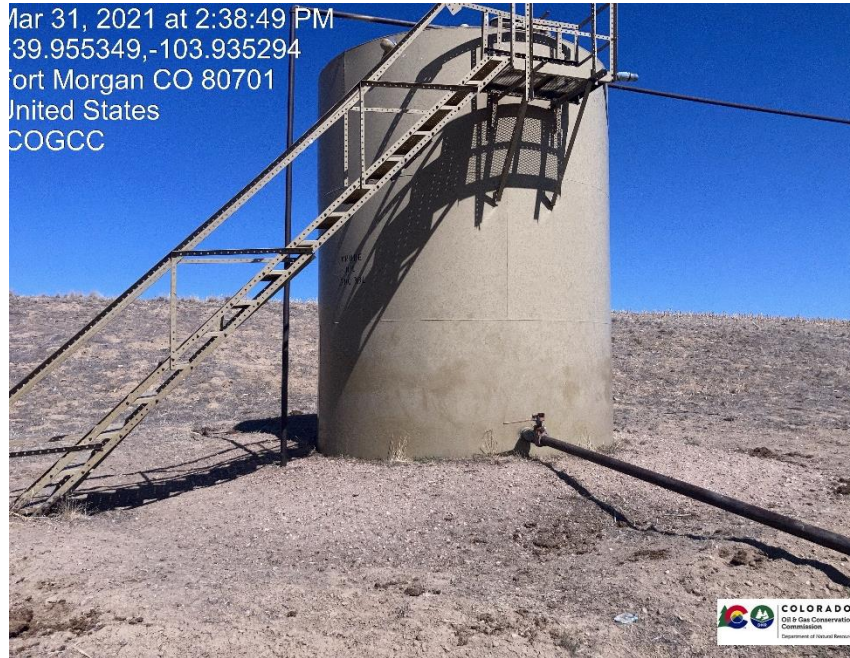
Pic 5 tank, berms need rebuilt, /no sign
