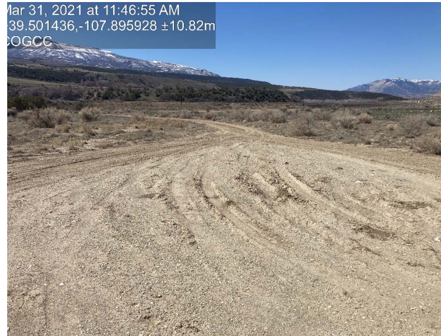
Lack of stabilization/ compaction
