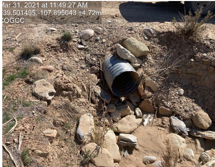
Culvert on access road needs maintained
