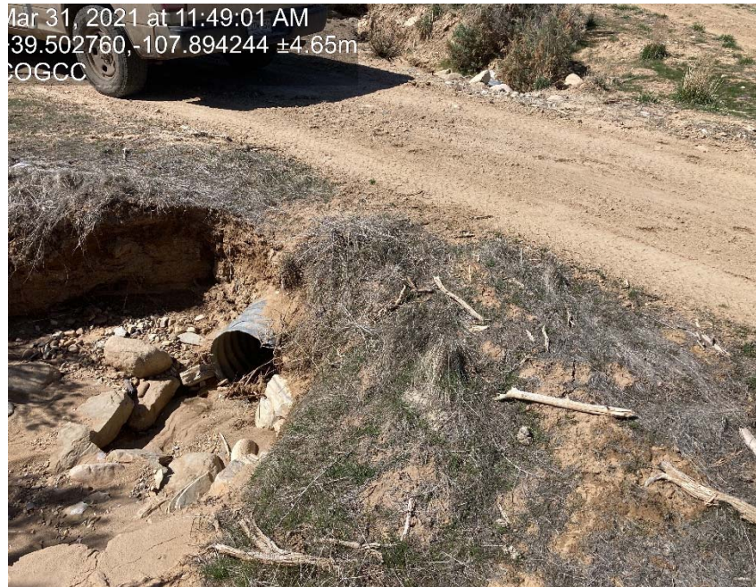
Culvert on access road needs maintained
