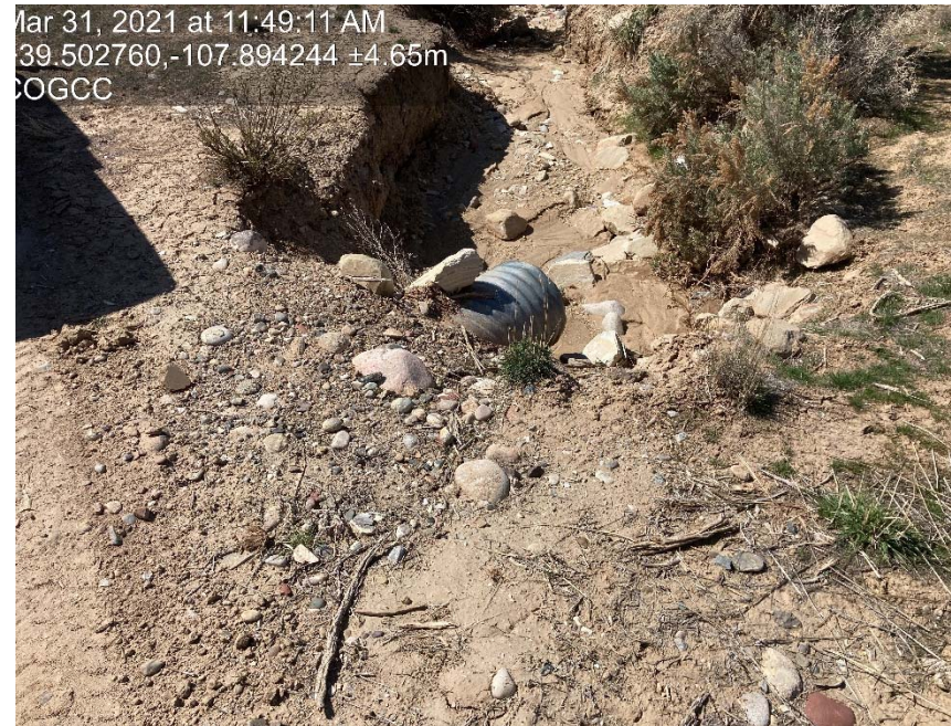
Culvert on access road needs maintained
