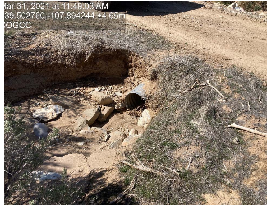
Culvert on access road needs maintained
