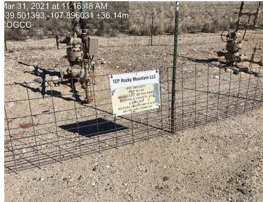
Signage is starting to fail
