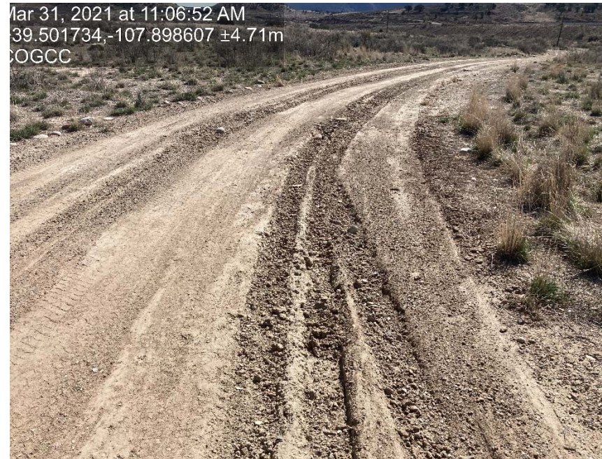
Lack of stabilization/compaction
