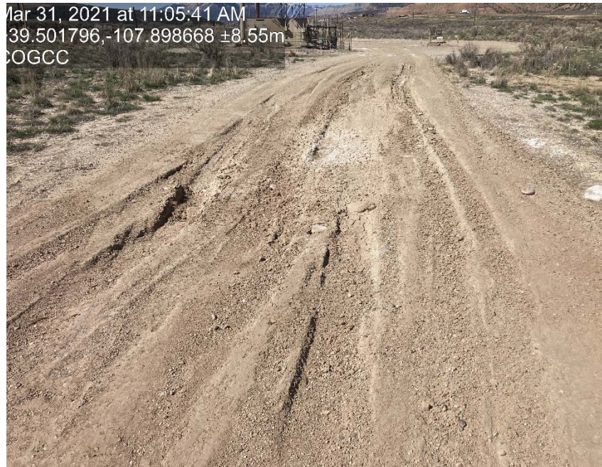
Lack of stabilization/compaction
