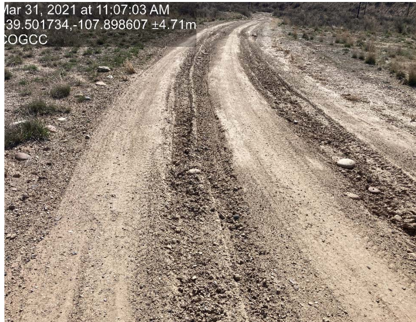
Lack of stabilization/compaction
