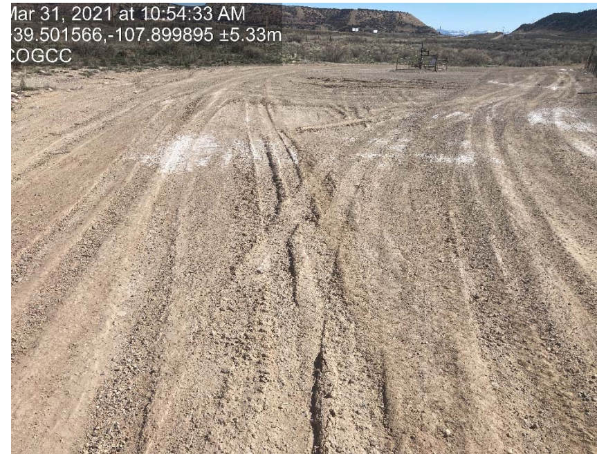
Lack of stabilization/compaction
