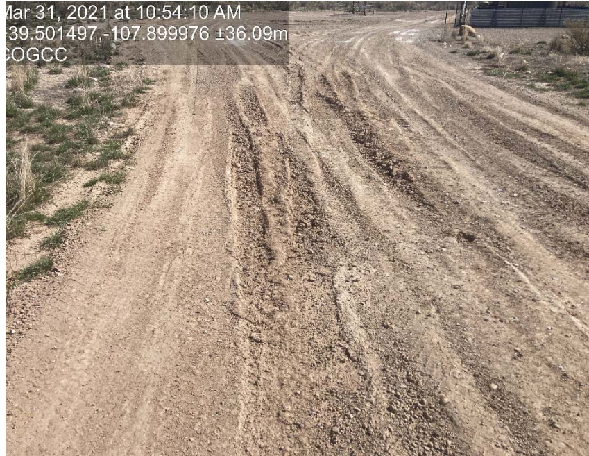
Lack of stabilization/compaction
