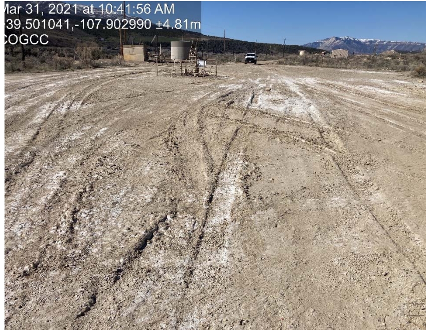
Lack of stabilization/compaction
