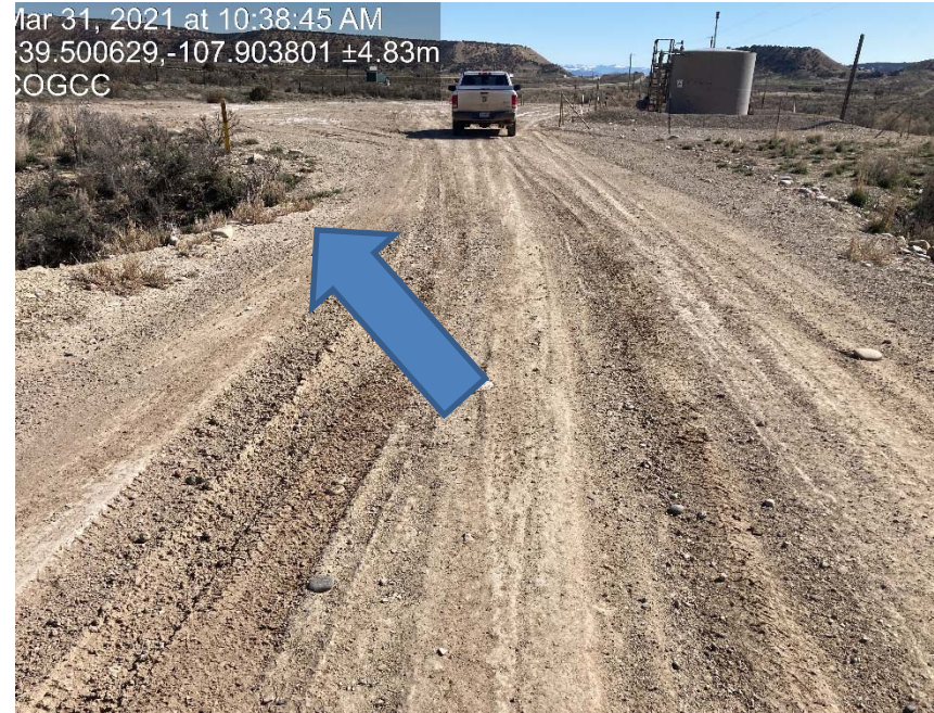
Entrance to location over culvert arrow is location of erosion
