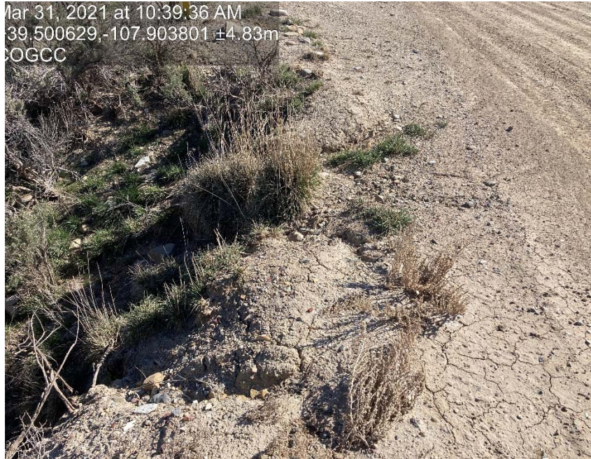
Erosion over culvert at entrance
