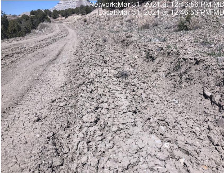
Photo #3359 Sediment has migrated into ditch
