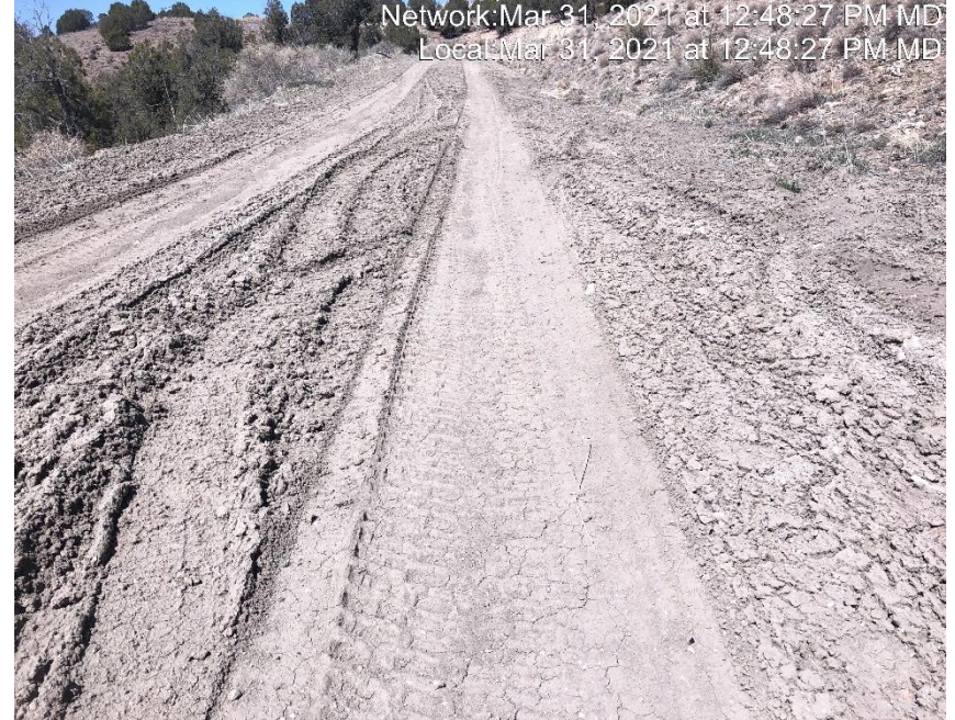
Photo #3360 Access road lacks stabilization.
