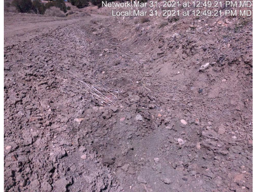
Photo #3361 Sediment has migrated into ditch
