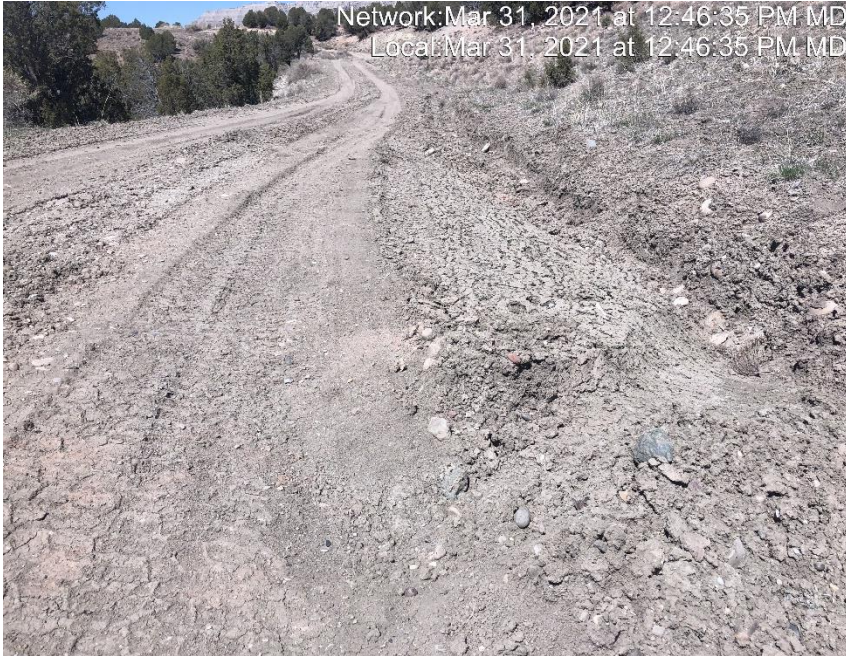
Photo #3358 Access road lacks stabilization.
