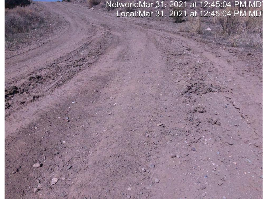
Photo #3357 Access road lacks stabilization.
