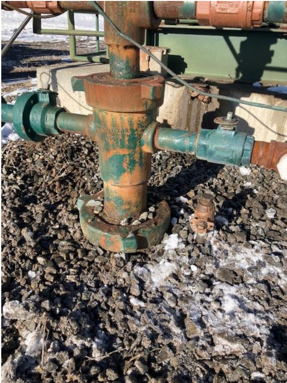
Bradenhead is plumbed to surface
