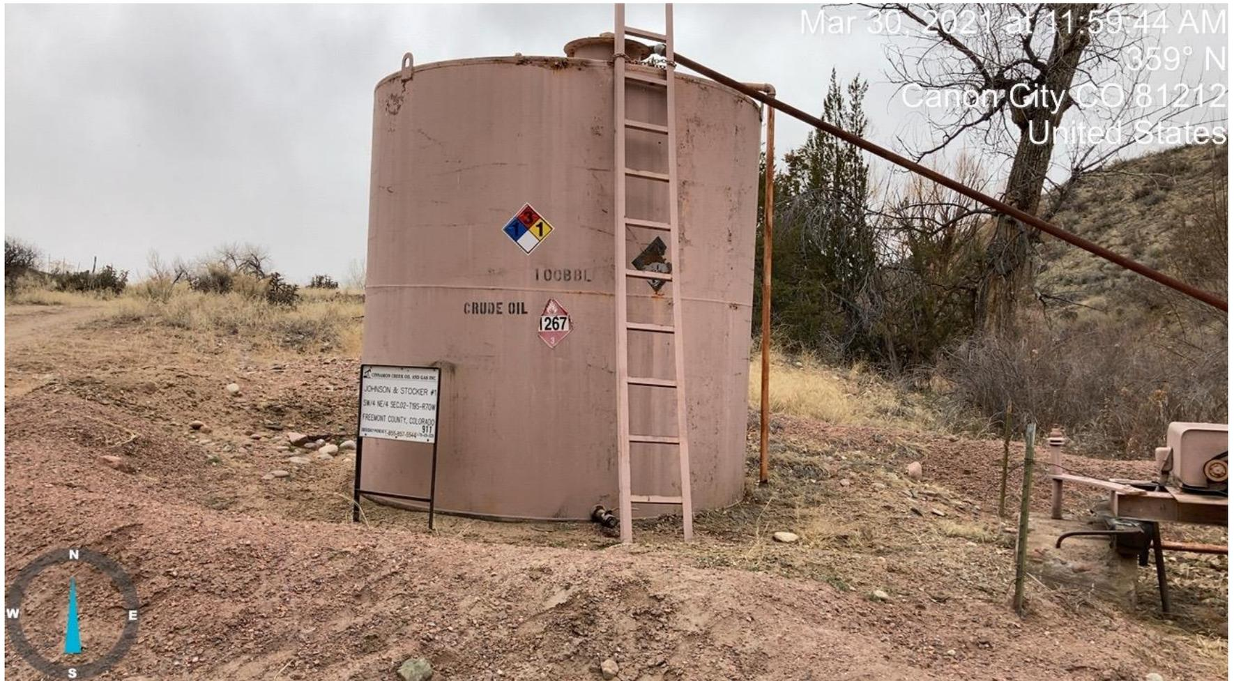
**PHOTO 5: WELL IS WITHIN A DESIGNATED FLOOD PLANE AND CRUDE OIL TANK HAS NO ANCHORING. Anchor equipment ensuring anchors are engineered to ensure the equipment will resist flotation, collapse, lateral movement, or subsidence per Rule 607. CA DATE 5-30-21.**
