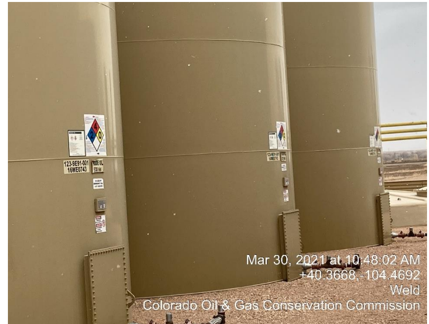
Photo #14 Weathered Capacity Label
