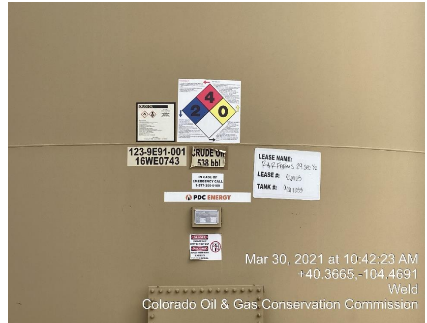
Photo #12 Weathered Capacity Label
