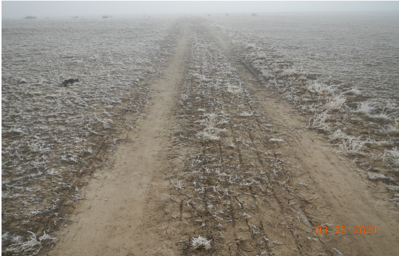
Photo 2. Facing east along the access road. It appears the a portion of the road was recently seeded however, the road is compacted. The road needs to be decompacted and reseeded.
