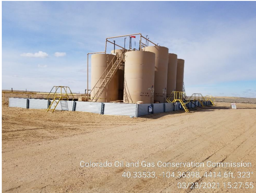
Photo 3 – Tank Battery
