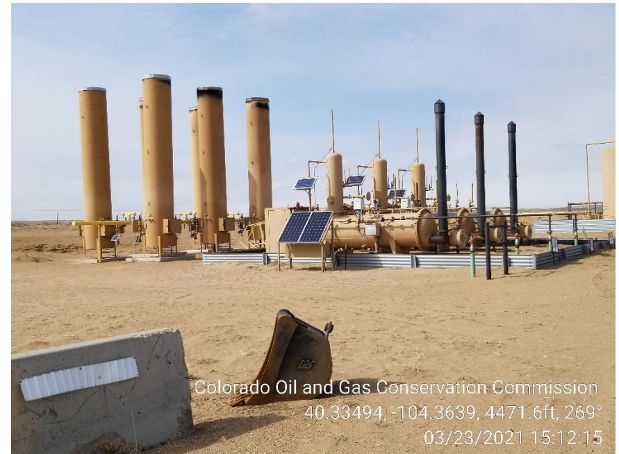
Photo 2 – Separators and ECDs
