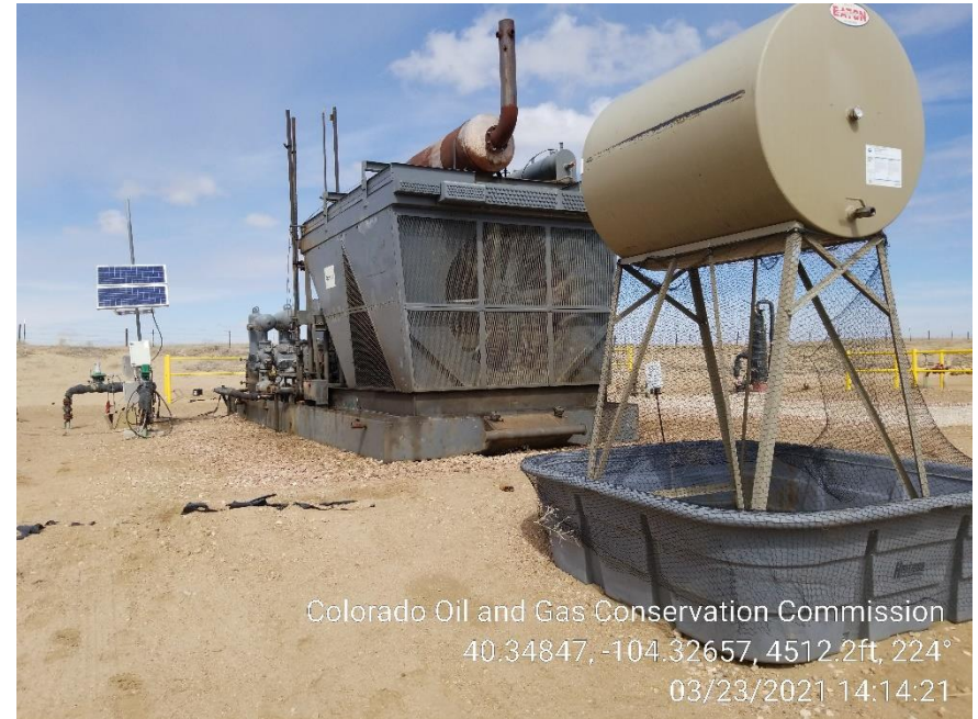
Photo 4 – Compressor – Day Tank now has Wildlife Netting
