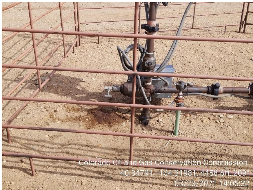
Photo 3 – 11-14-3HNB Wellhead – Stained Soil
