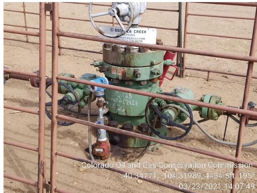
Photo 2 – A-E-3HNB Wellhead – Stained Soil
